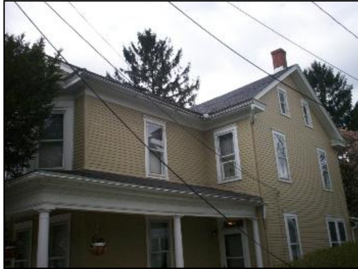
1. Upper gutter inside corner
