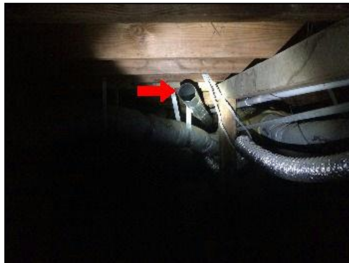
1. Poor slope / terminating in crawlspace
