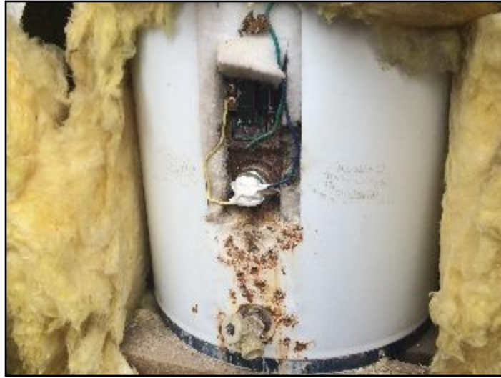
2. Evidence of leaking at bottom element
