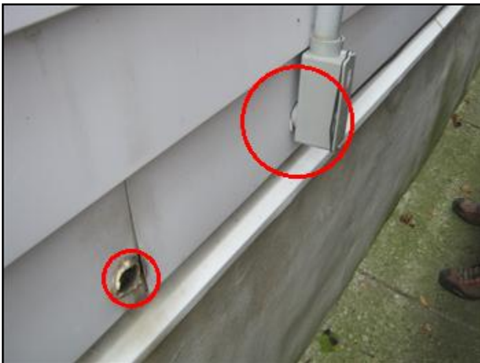
seal gaps to prevent water entry
