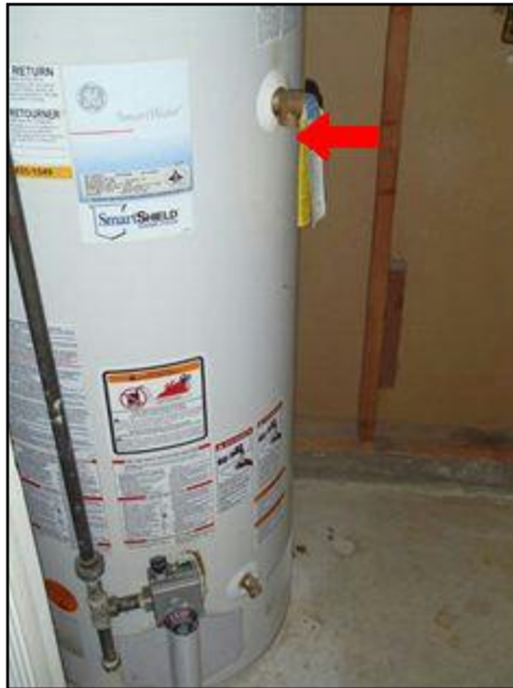
Discharge tube missing
