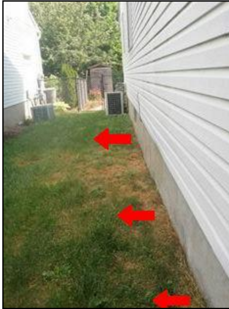
27. Improper slope
