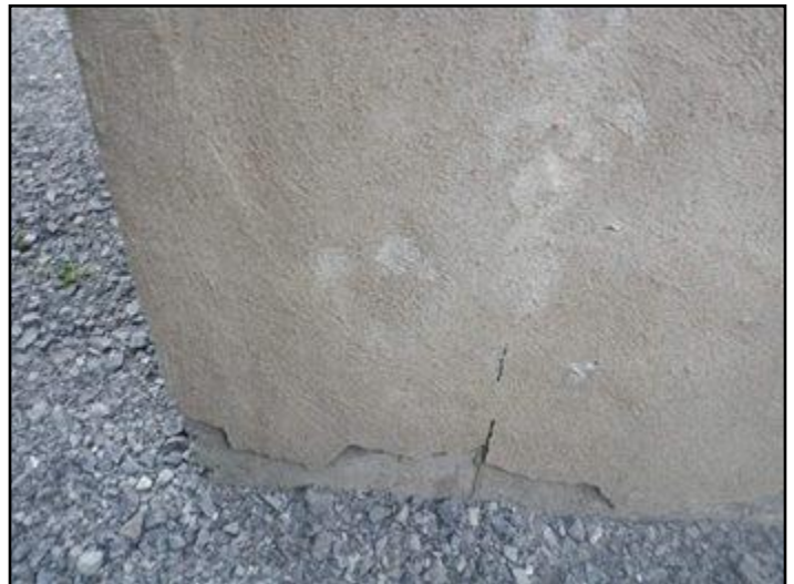
38. Parging damaged or missing
