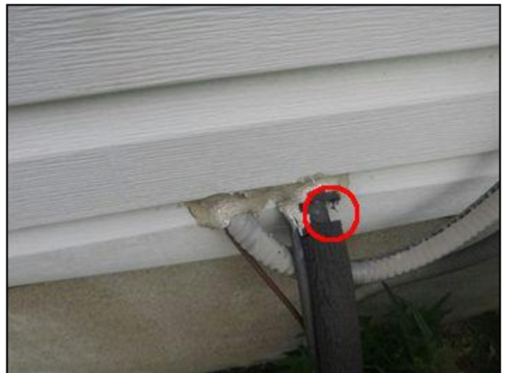
59. Missing insulation
