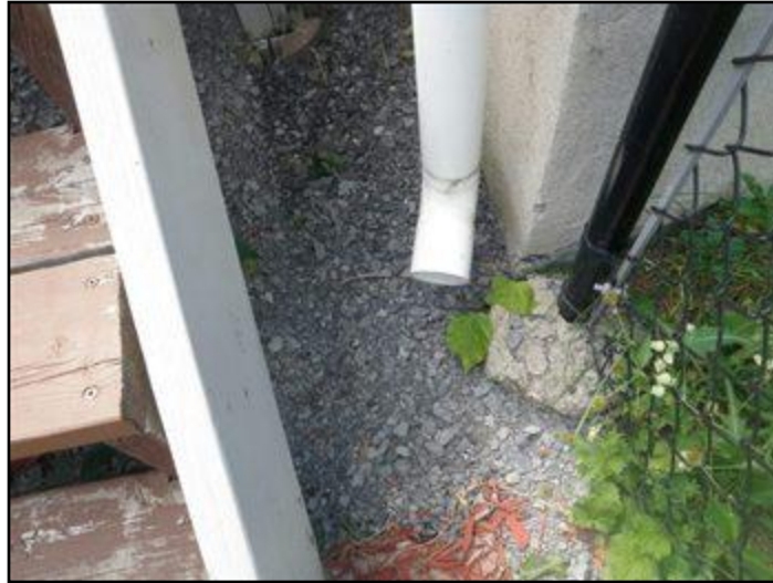
12. Downspouts end too close to building
