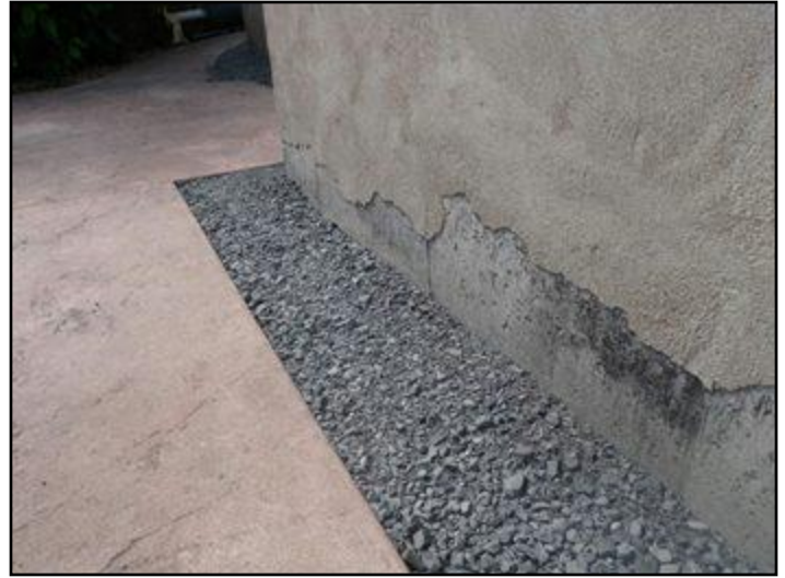
40. Parging damaged or missing
