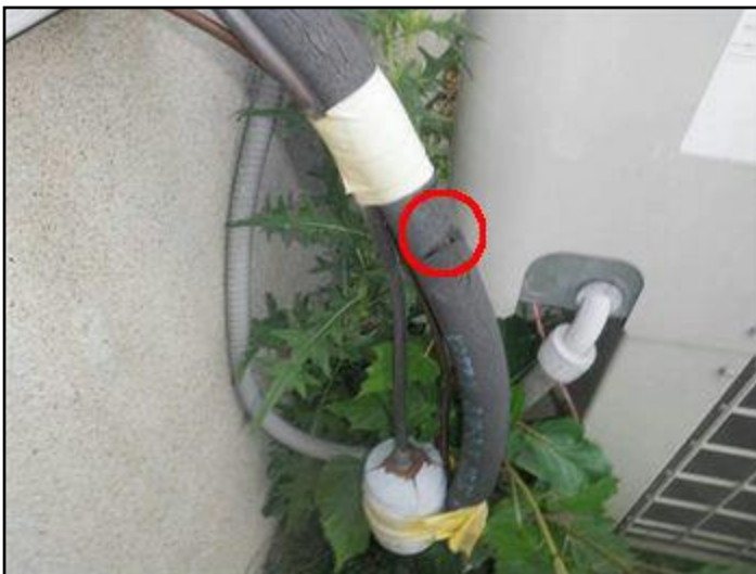
58. Missing insulation
