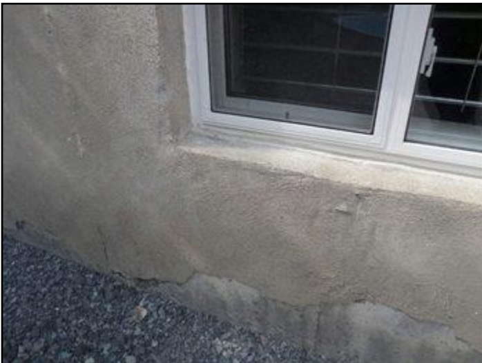
37. Parging damaged or missing
