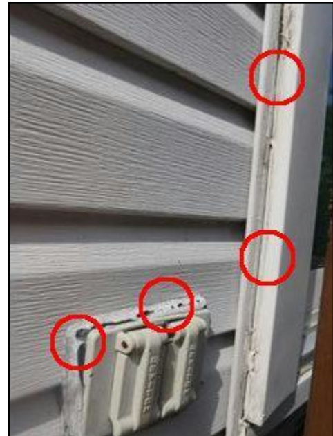
14. Caulking missing or ineffective
