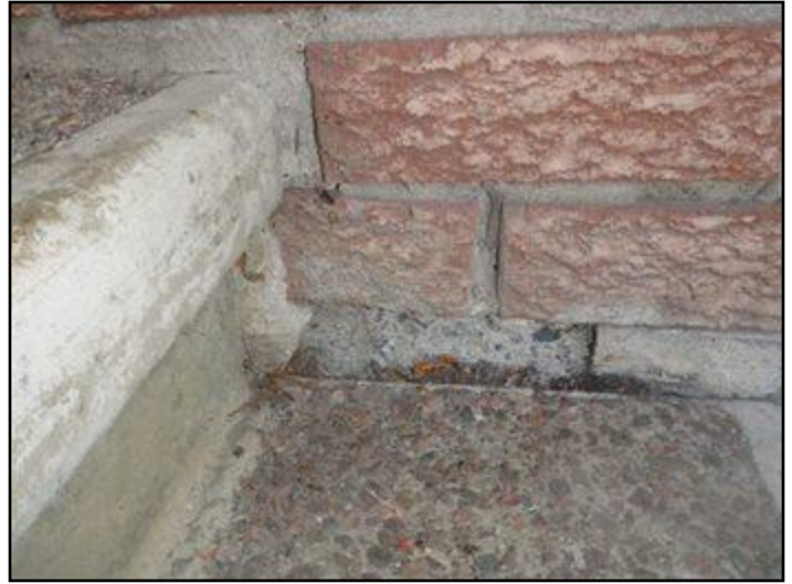
36. Parging damaged or missing
