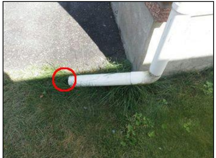
11. Downspouts end too close to building
