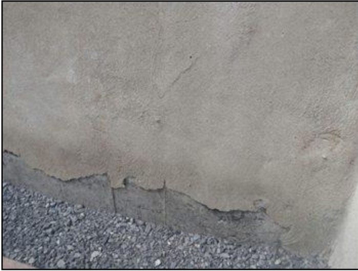
39. Parging damaged or missing
