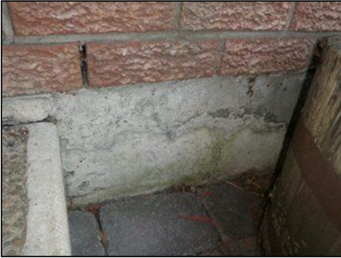
35. Parging damaged or missing
