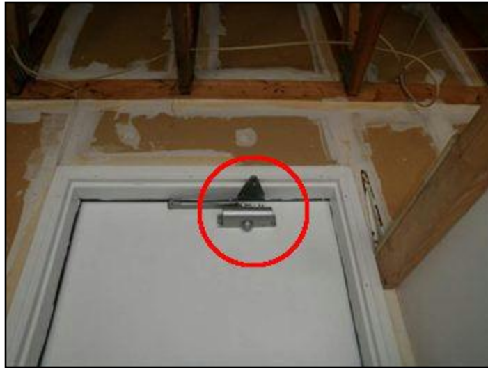
32. Self Closer disconnected
