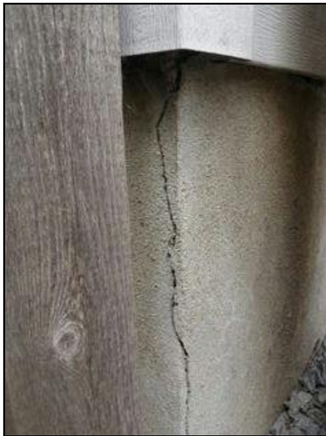
41. Parging damaged or missing
