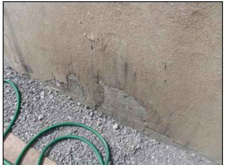
42. Parging damaged or missing
