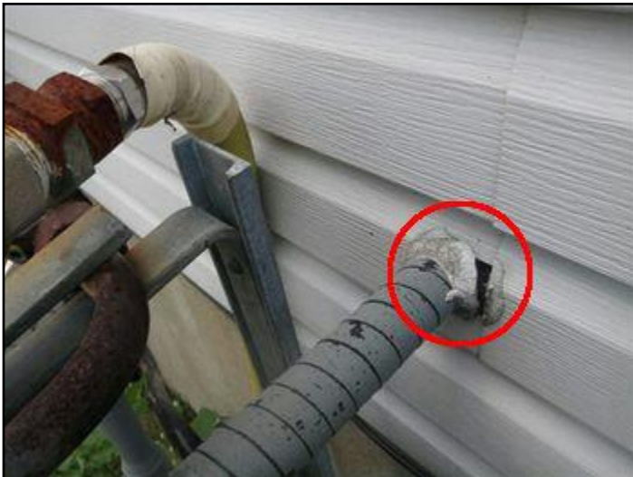
13. Caulking missing or ineffective
