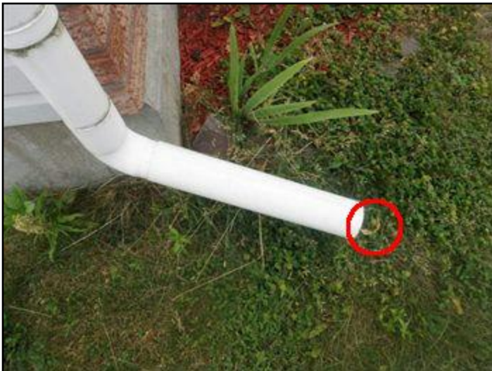
10. Downspouts end too close to building
