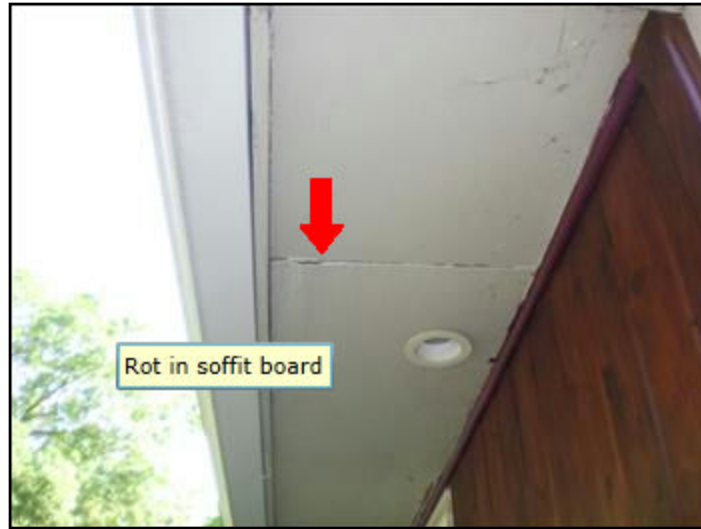
4. Rot or insect damage
