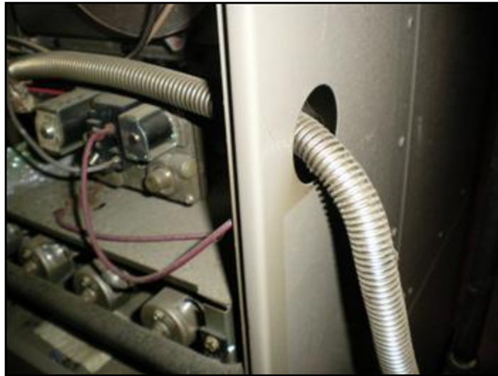
26. Inappropriate materials
