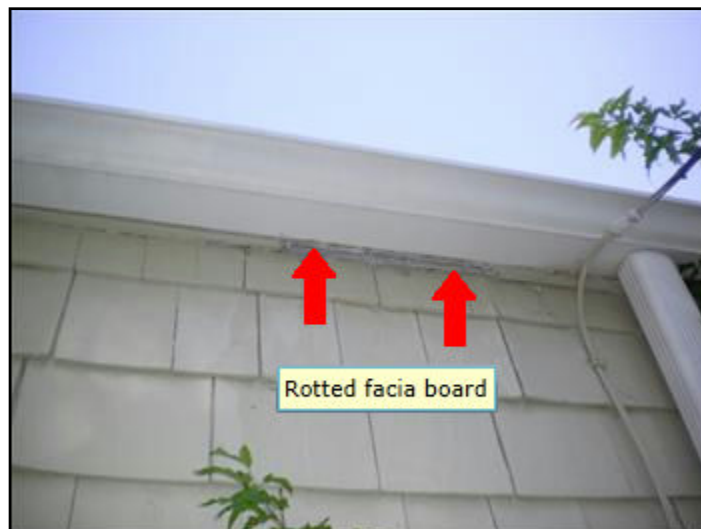
5. Rot or insect damage
