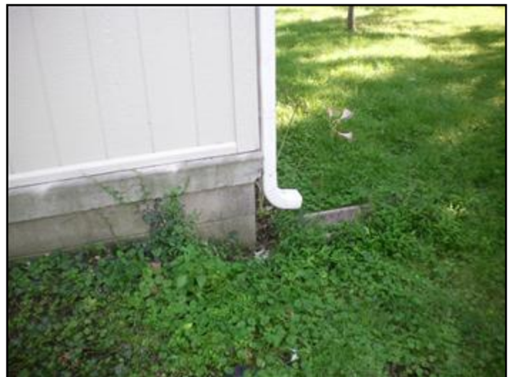
2. Should discharge 6ft. from home
