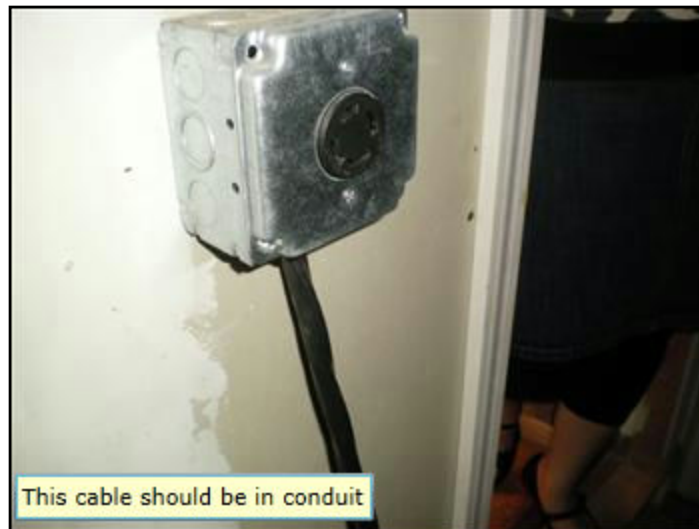
18. Exposed on walls or ceilings
