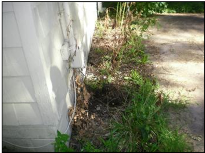
10. Improper slope
