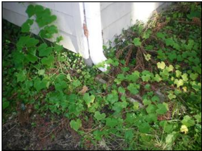
3. Should discharge 6ft. from home
