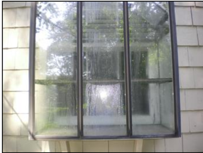
37. Lost seal on double or triple glazing
