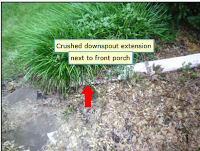
1. Should discharge 6ft. from home
