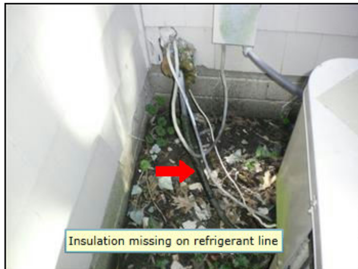
29. Missing insulation
