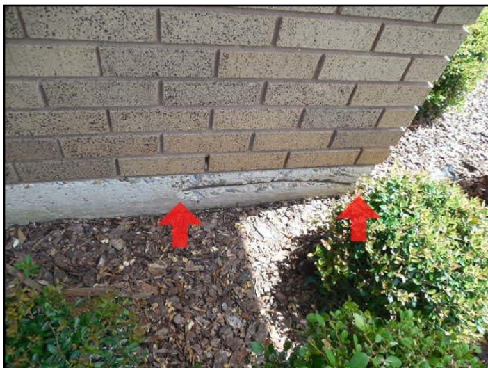
21. Typical minor cracks
