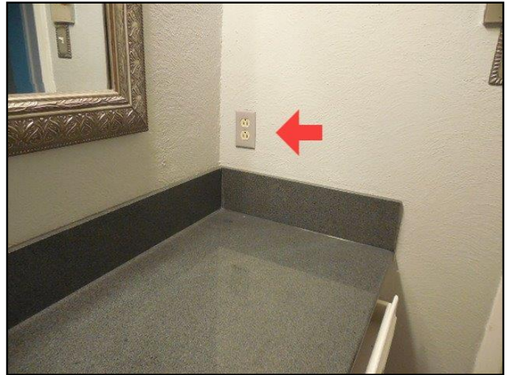
26. No GFCI - bathroom
