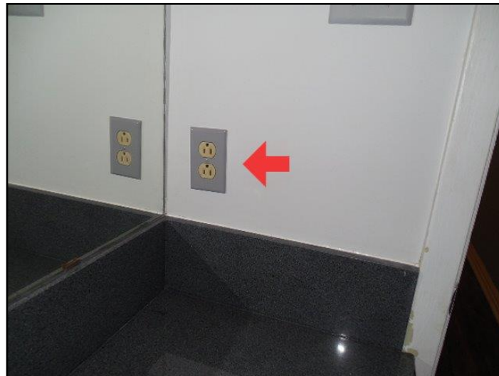
30. No GFI (Ground Fault Interrupter)
