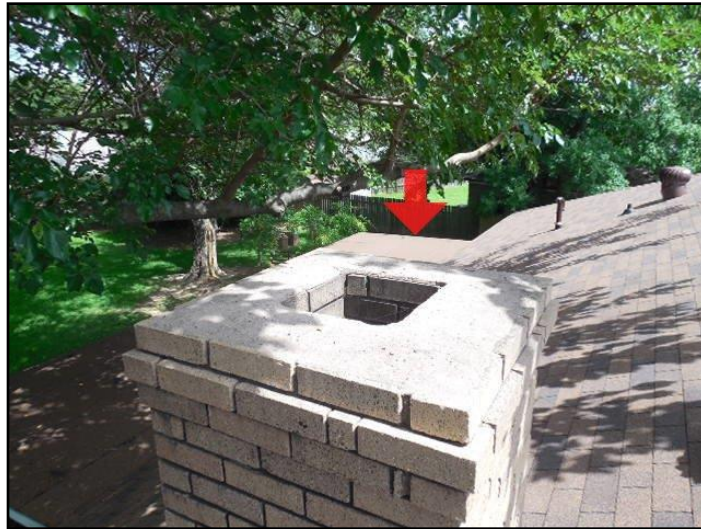
31. Chimney cap needed
