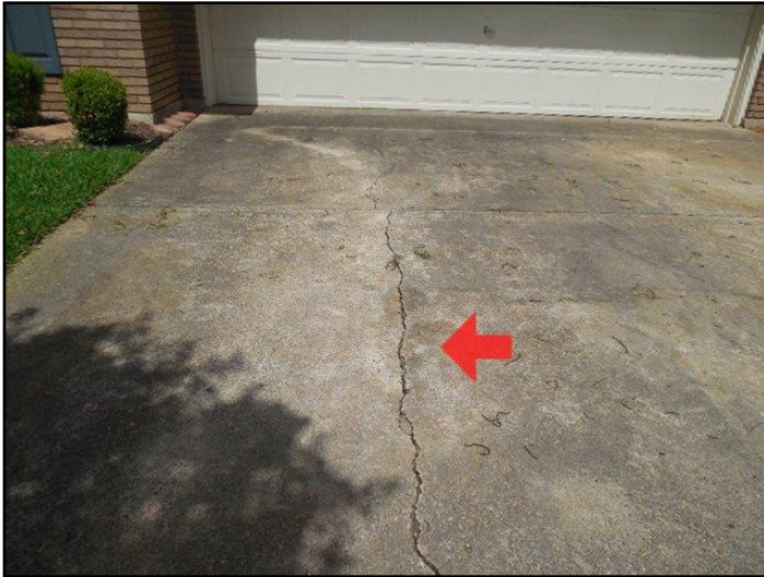
7. Cracked or damaged surfaces
