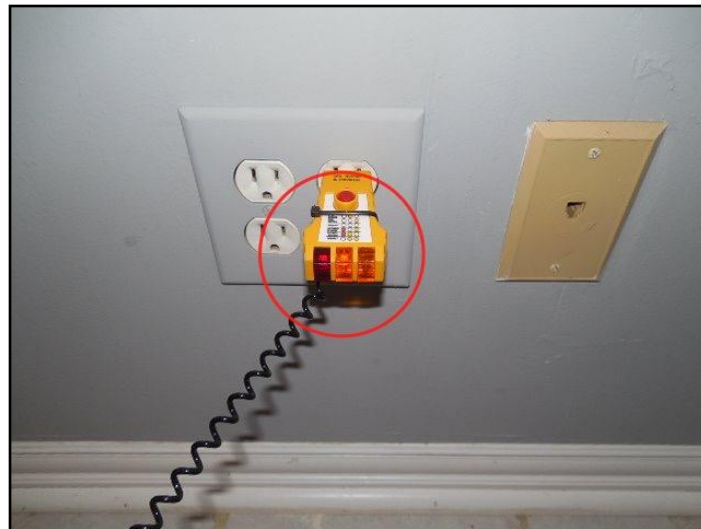
27. Reversed polarity
