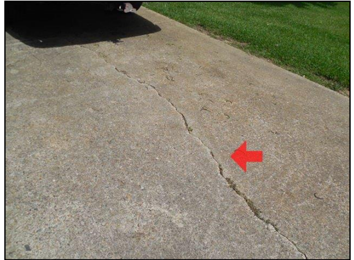
8. Cracked or damaged surfaces
