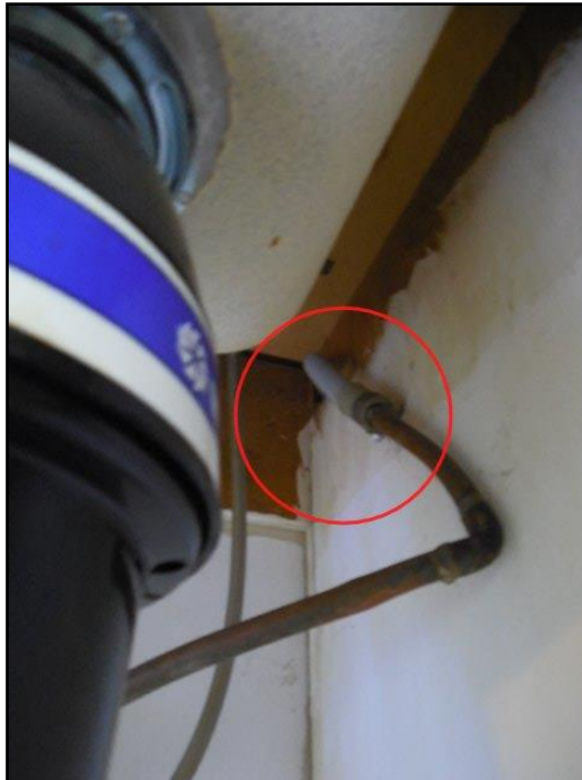
35. Backflow prevention missing
