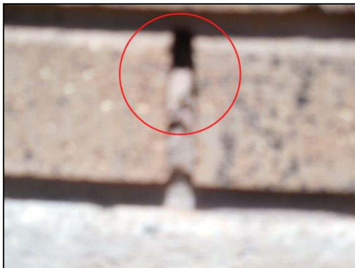
4. Missing, ineffective weep holes or flashings
