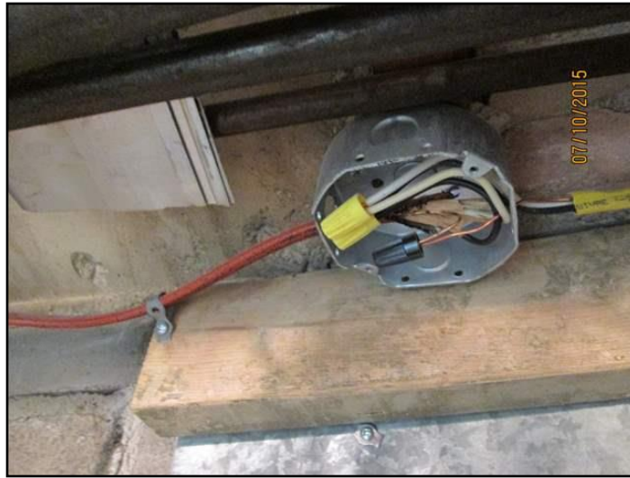
Cover Plate(s) - missing
