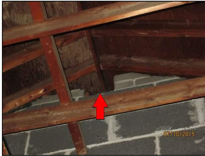
Gas proofing inadequate between Garage and...
