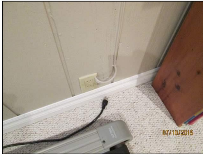
Surface mounted wiring - unprotected
