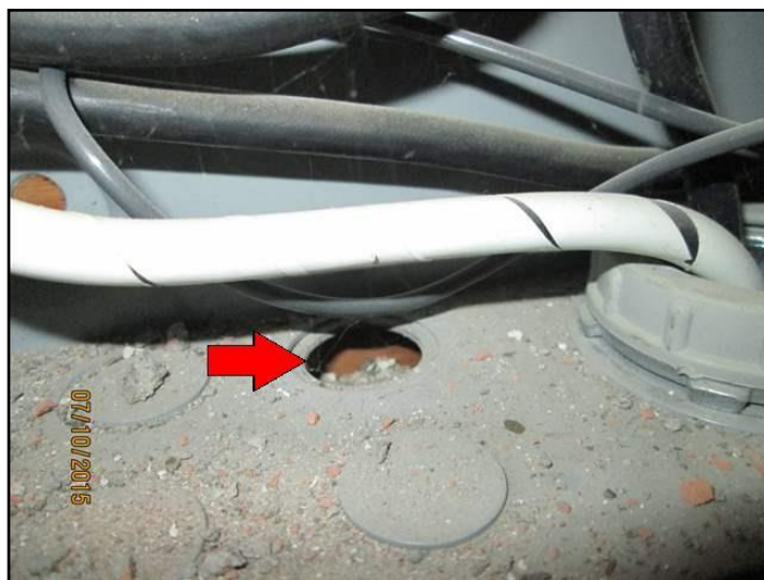
Unprotected openings
