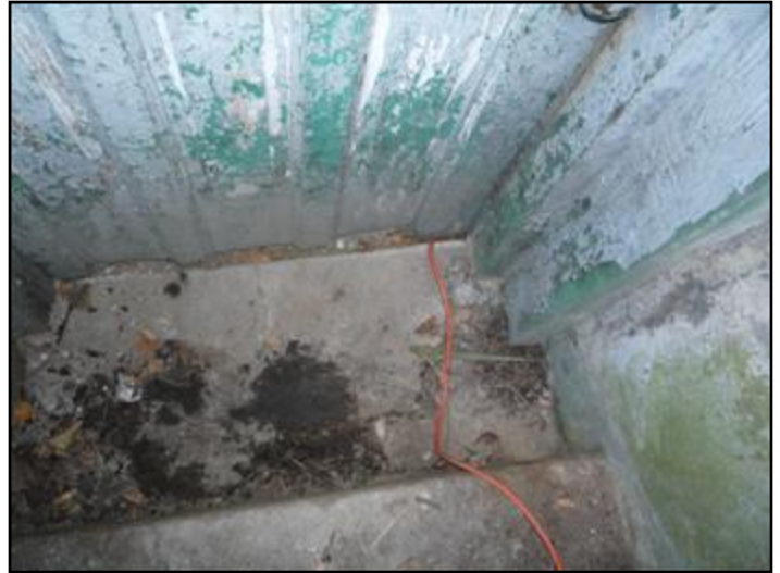
provide drain and threshold
