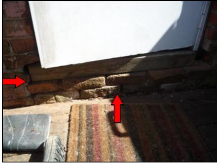
Mortar deterioration
