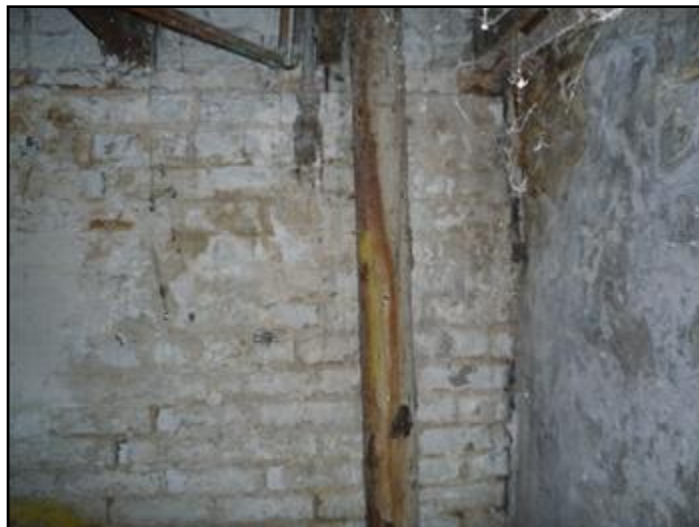
old stack leaks
