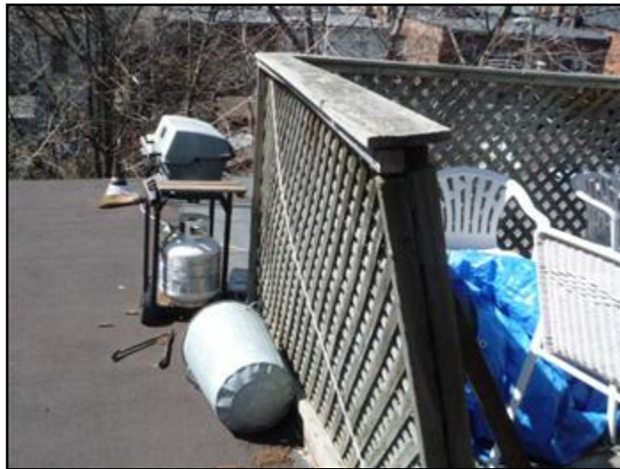
loose and missing rail
