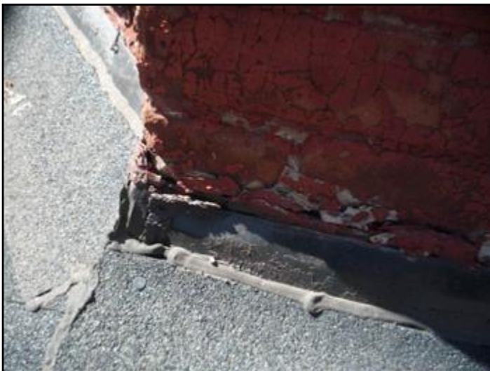
poor seal at flashing
