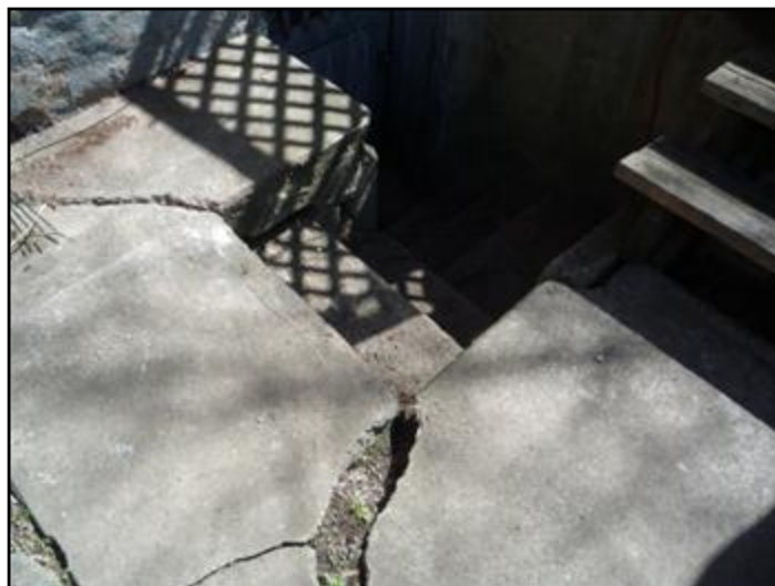
repair cracks and provide guardrail
