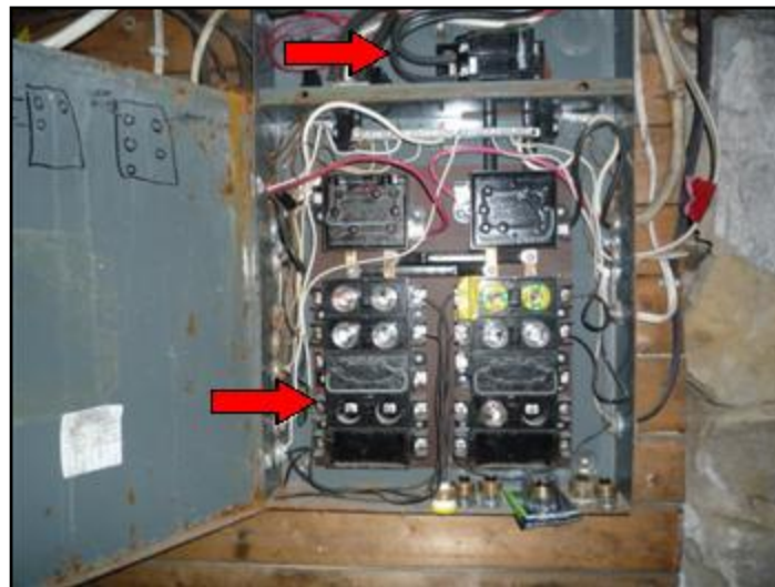
unprotected openings
