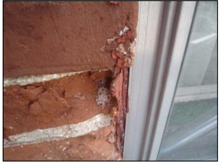
spalling bricks
