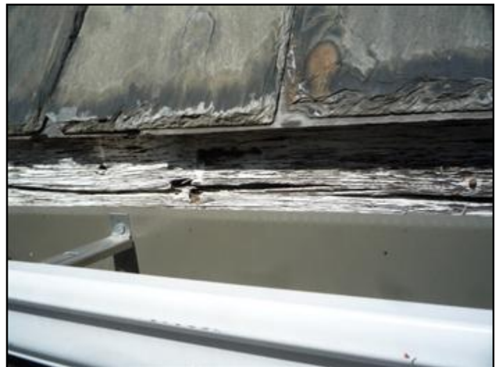
provide drip edges
