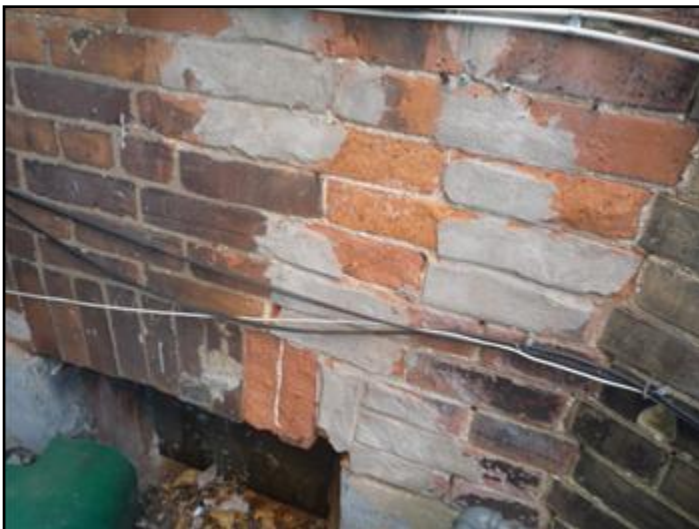
water damage
