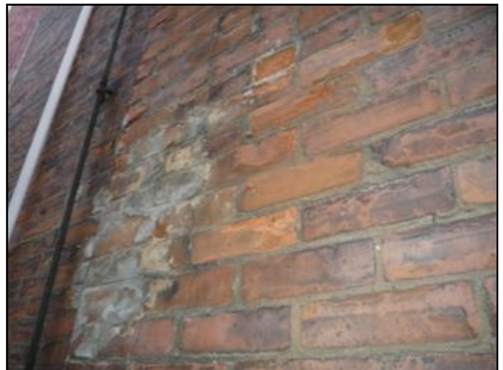
spalling chimney
