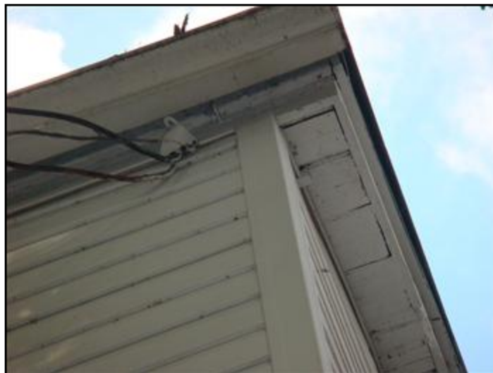
12. cable covered with siding
