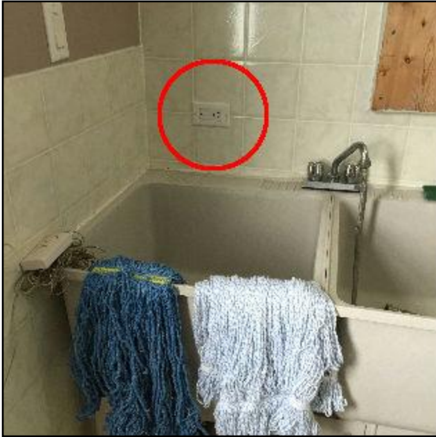
22. Ground Fault Interrupter (GFI) needed
