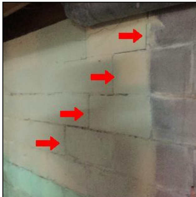
16. Typical minor cracks
