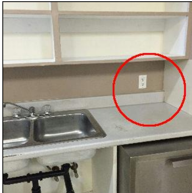
24. Ground Fault Interrupter (GFI) needed
