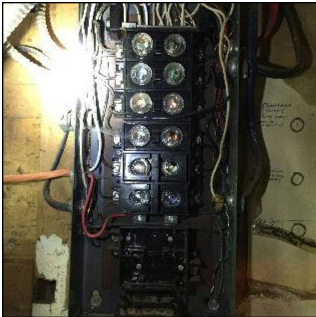
18. Unprotected openings
