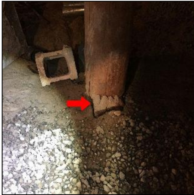
17. Wood/soil contact
