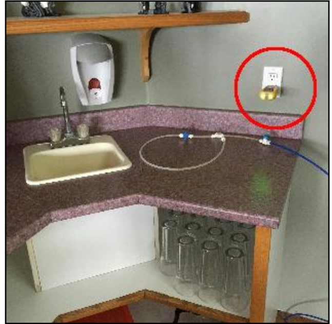
23. Ground Fault Interrupter (GFI) needed
