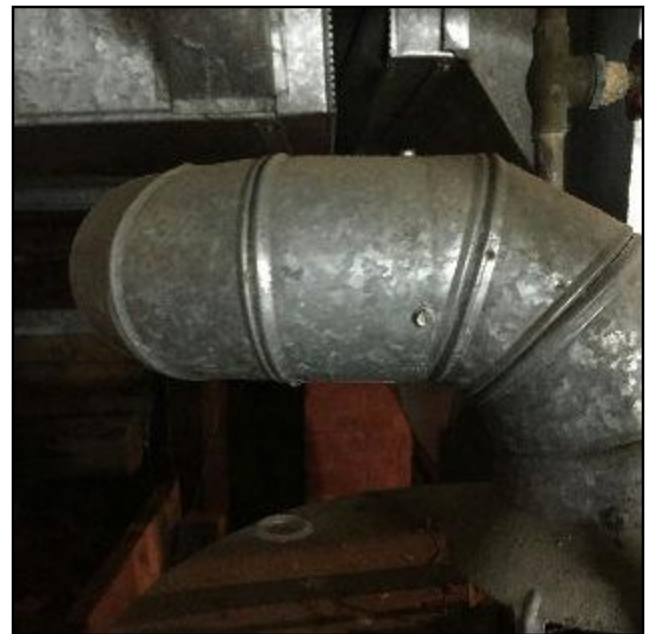
28. Vent connector extends too far into chimney
