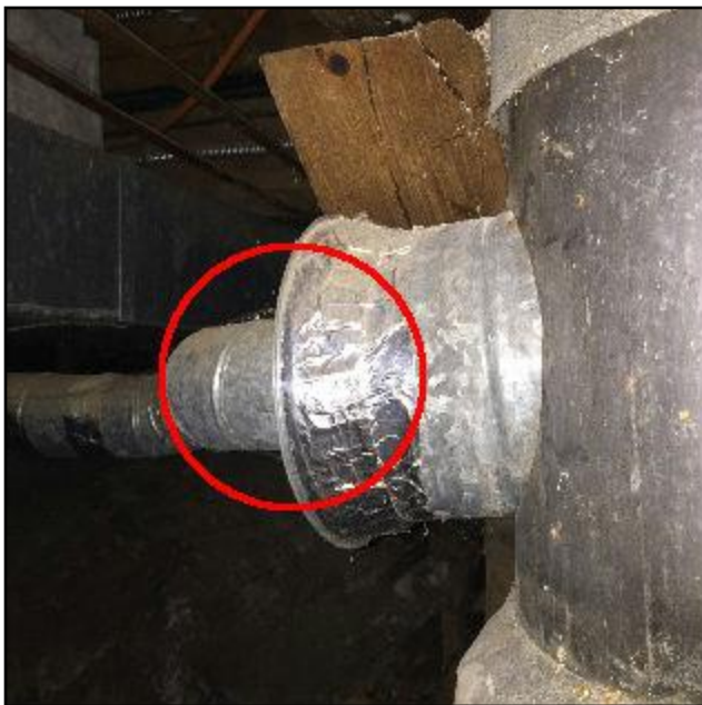
27. Vent connector extends too far into chimney
