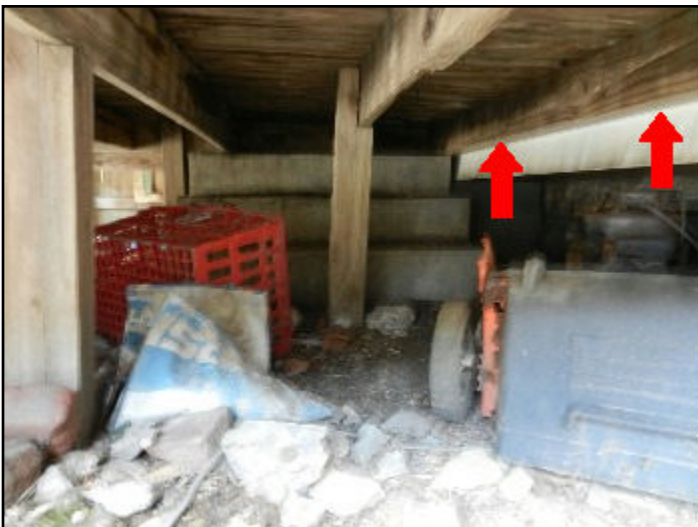
17. Ledger board not bolted to house frame
