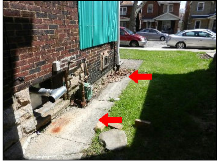
23. Improper slope
