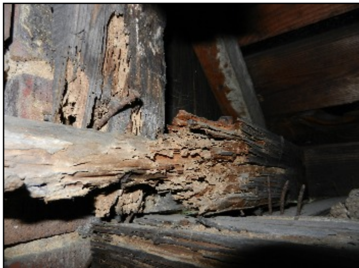
27. Extensive termite damage in back-left corner.
