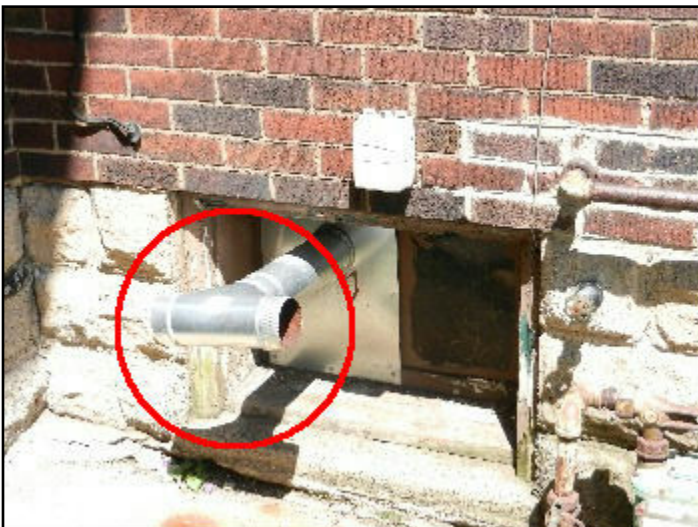
37. Boiler vent termination outside.
