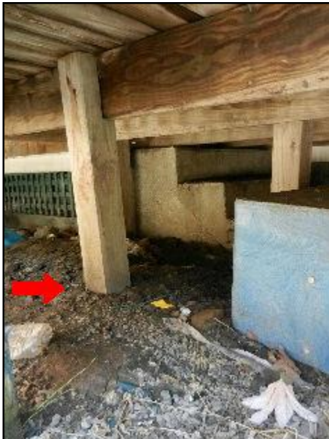
15. Posts in contact with earth
