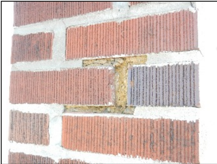
54. Thin pointing of bricks on chimney.
