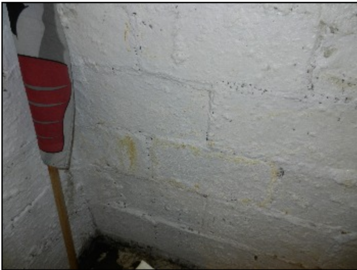
75. Dampness on floor or walls
