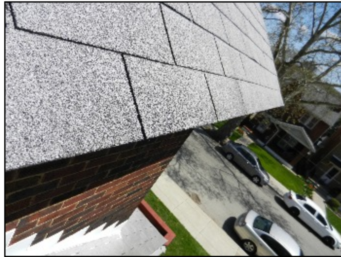
8. Missing gutter on garage.
