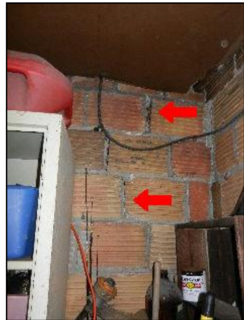
31. Crack/gap in mortar joints
