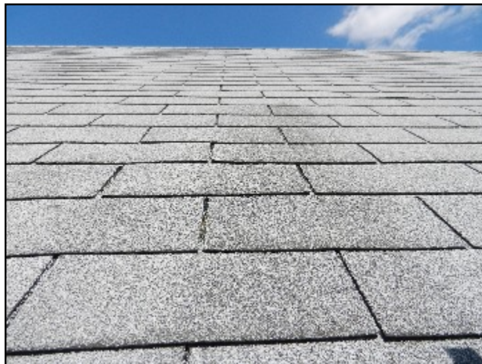
3. Some mineral loss on shingles.
