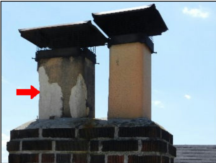
50. Spalling chimney liner
