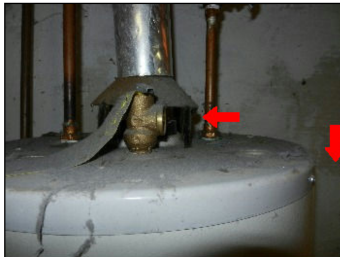
59. Discharge tube missing
