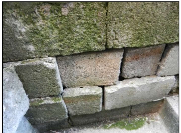
13. Blocks are loose, shifting
