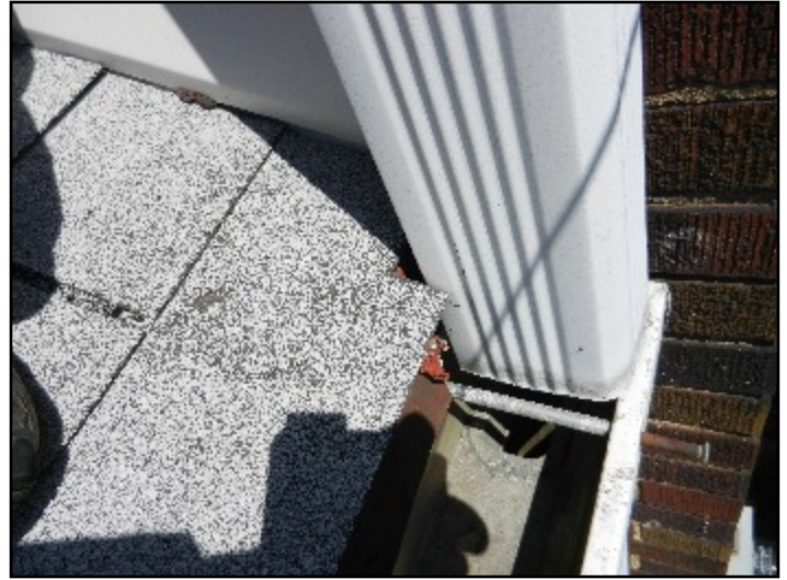
10. Downspouts to back porch roof gutter.
