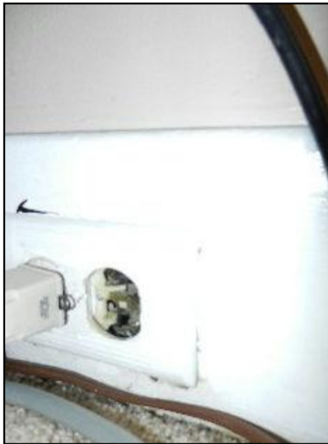
36. Damaged outlet
