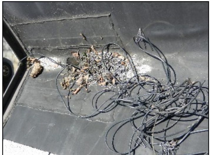
2. Valley detail--keep clear of debris
