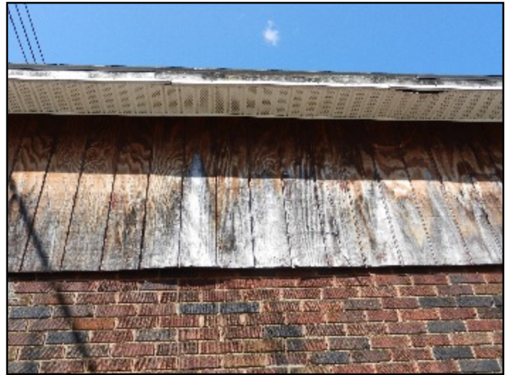
29. Wood siding warping, in need of paint
