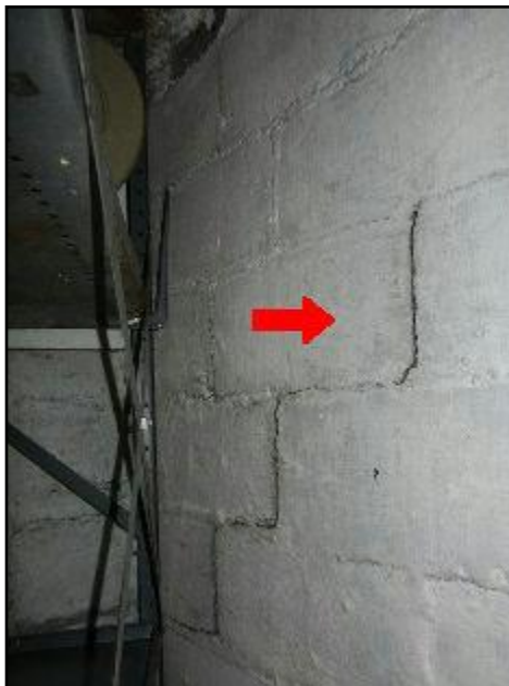
32. Typical minor cracks
