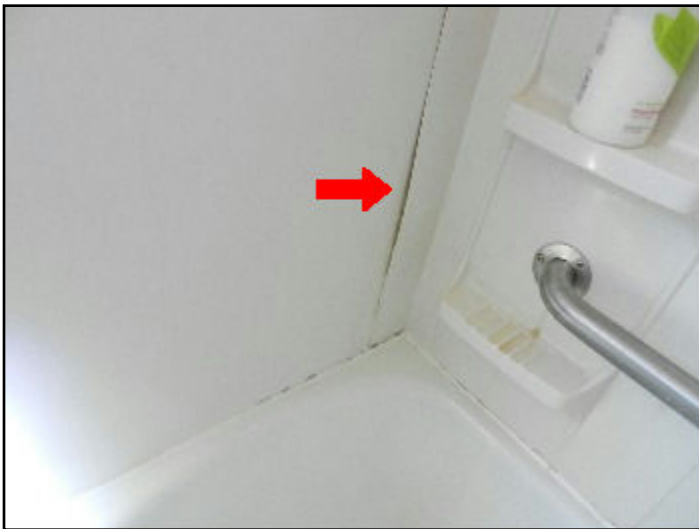
66. Not smooth, impervious or water resistant
