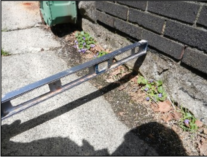
22. Improper slope
