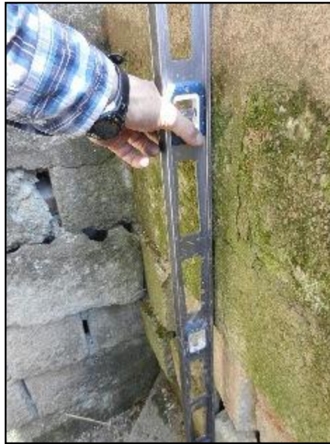
14. Walls cracking, leaning, bowing or spalling
