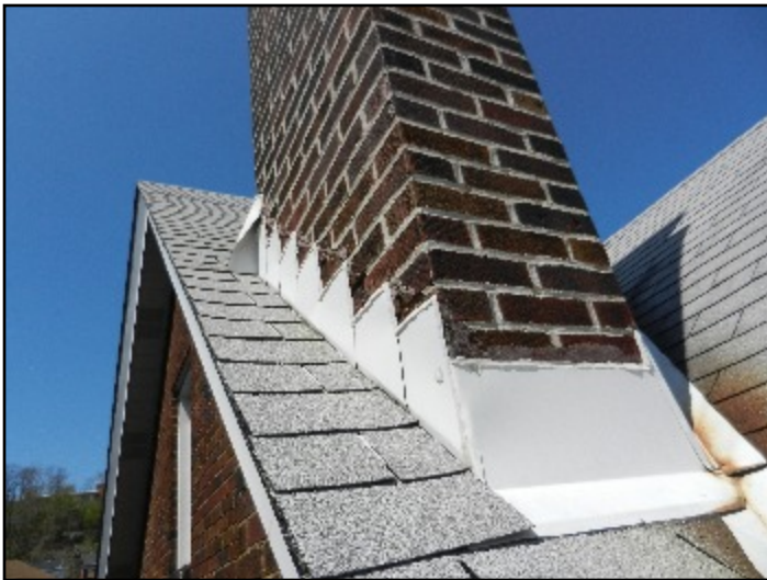
6. Not let into mortar joints
