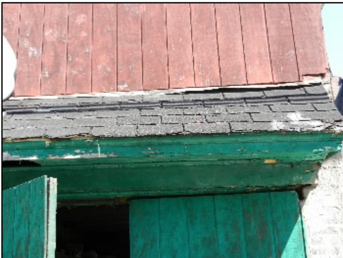
24. Over hang roof shingles deteriorated.
