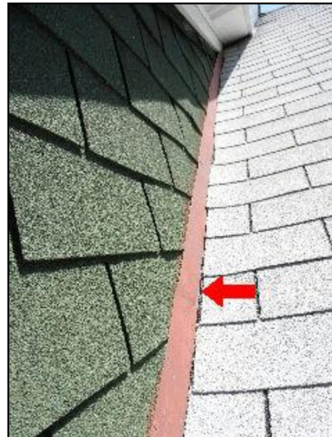
5. Missing cap flashings at rear dormer
