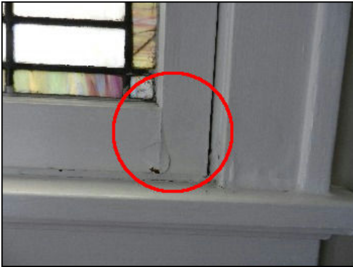
70. Sash cracked.
