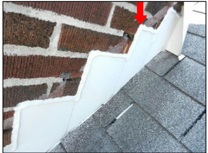
7. Not let into mortar joints
