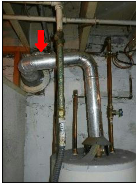
60. Vent connector slopes down.
