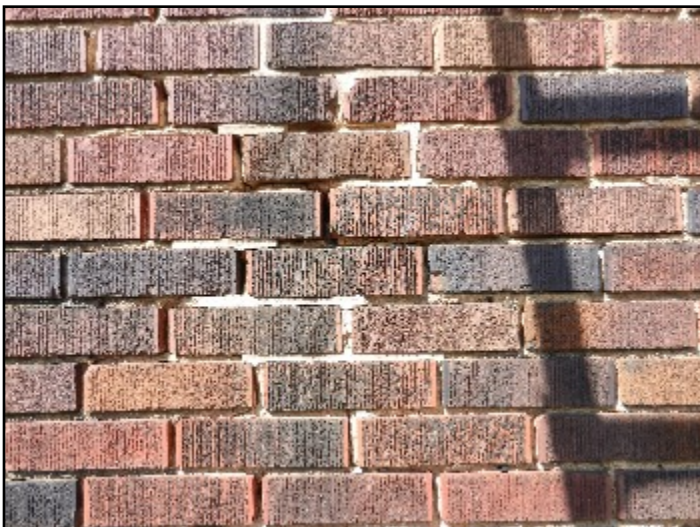
26. Mortar deterioration on garage wall.
