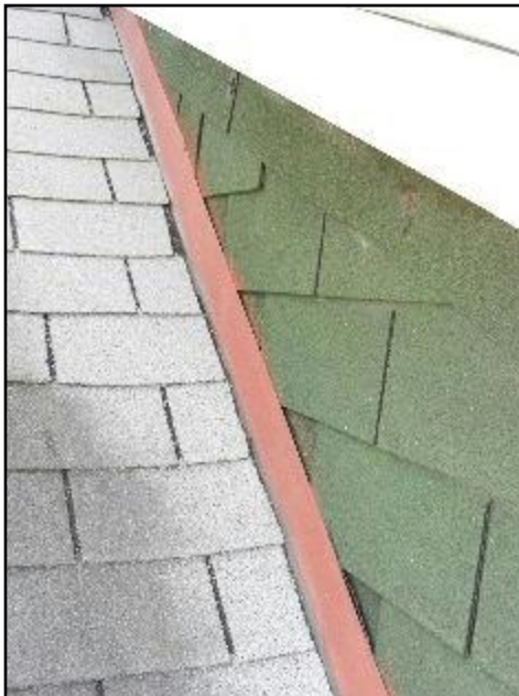
4. Missing base or cap flashings
