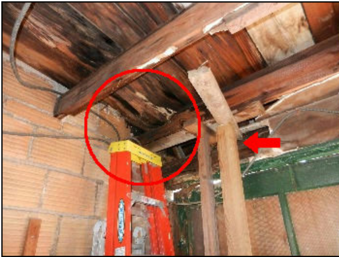
28. Damage to framing, posts holding up corner.
