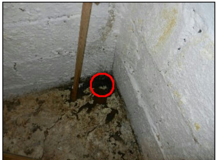
78. Dampness on floor or walls
