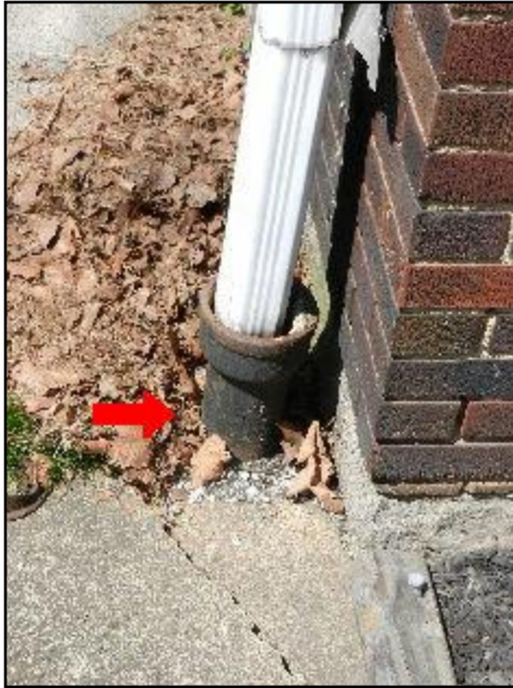
9. Downspouts discharging below grade
