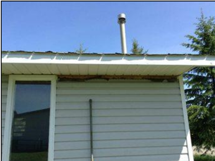
13. Garage wall missing siding
