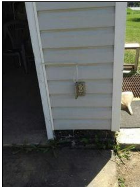
27. No GFI (Ground Fault Interrupter)
