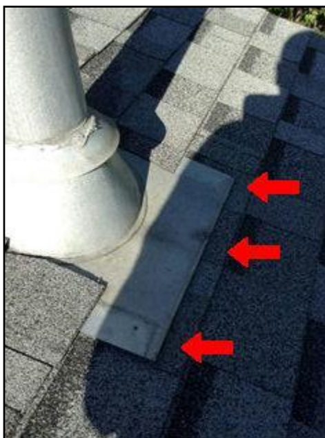
3. Exposed, missing fasteners
