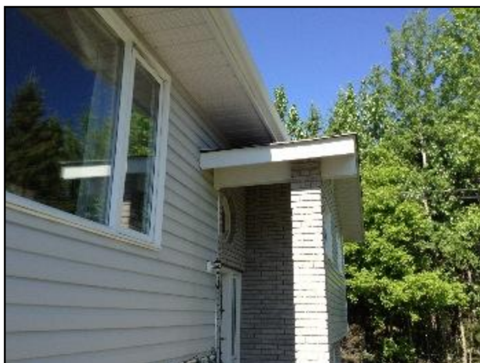
18. No gutter or downspout
