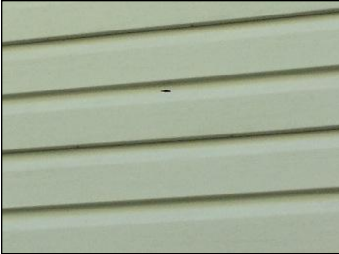
4. Minor Mechanical Damage
