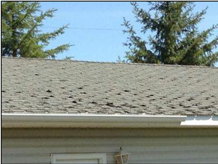
11. Garage shingles require replacement
