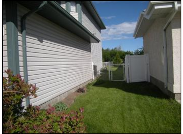
5. Right side yard.
