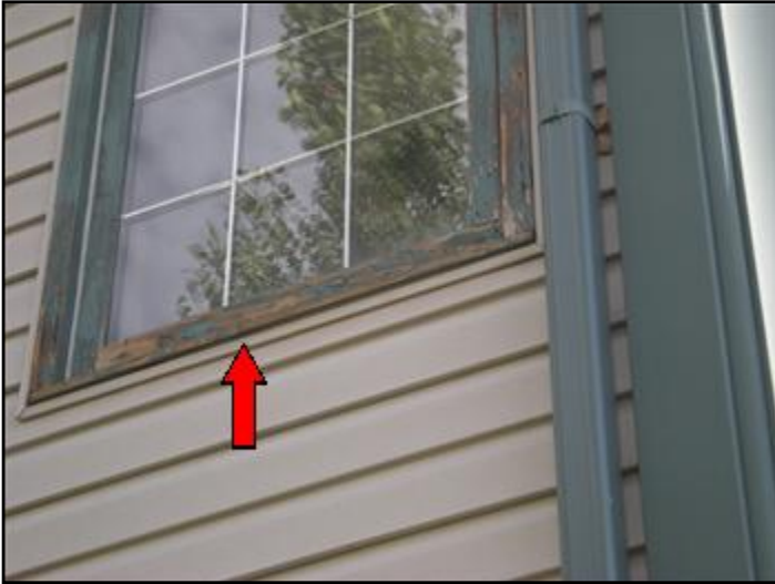
16. left side second storey.
