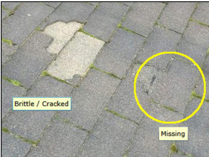
3. Asphalt shingles
