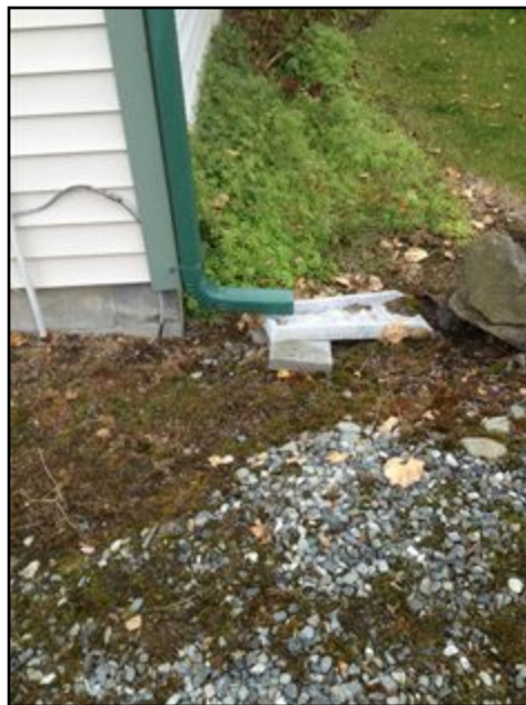
6. Downspouts end too close to building
