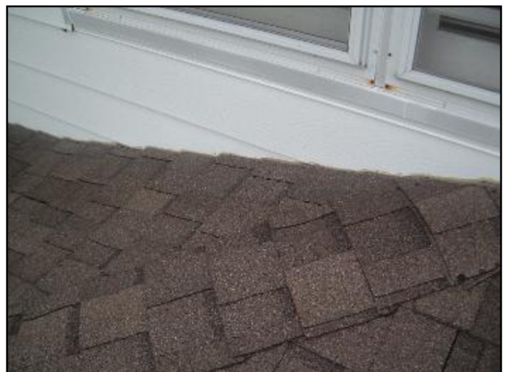
2. missing flashing
