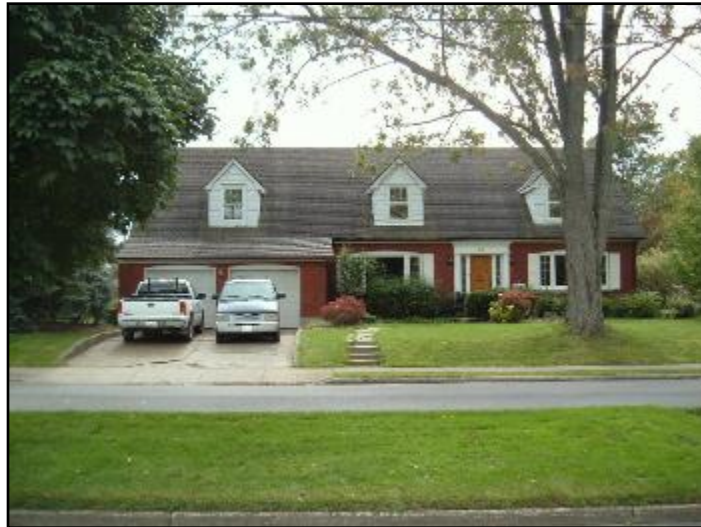
3. Dormers need gutters
