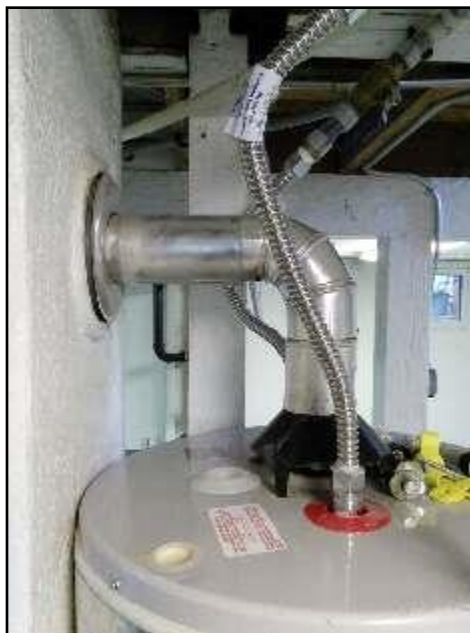
32. Poor slope
