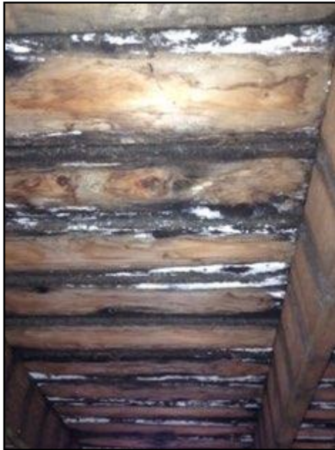
15. Rot or insect damage
