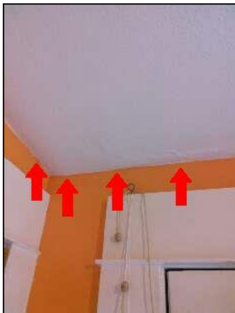
33. Water damage
