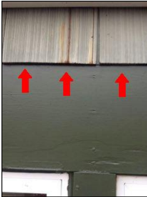
8. Flashings missing
