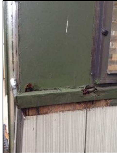
7. Rot or insect damage
