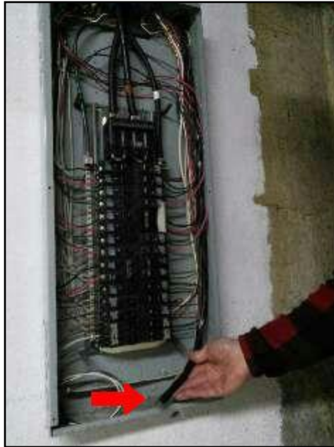
24. Abandoned wires in panel
