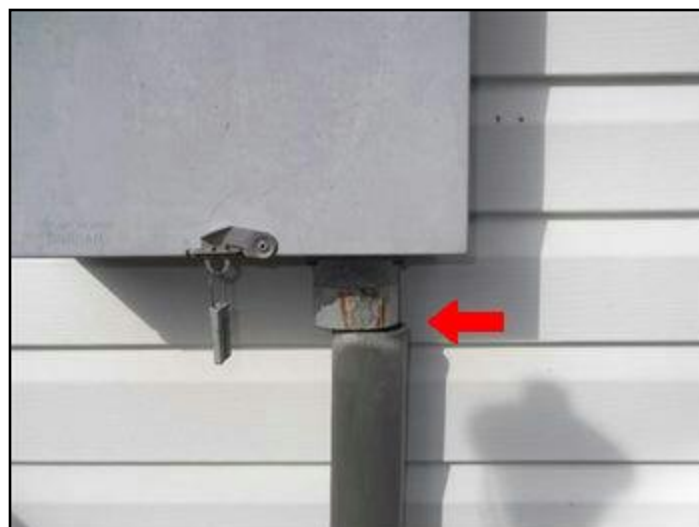
22. Supply to meter base- conduit not secure
