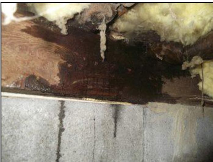
34. leaking pipe under kitchen
