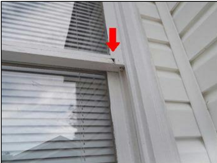
43. Water damage
