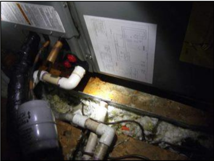
30. Air handler pan and drains
