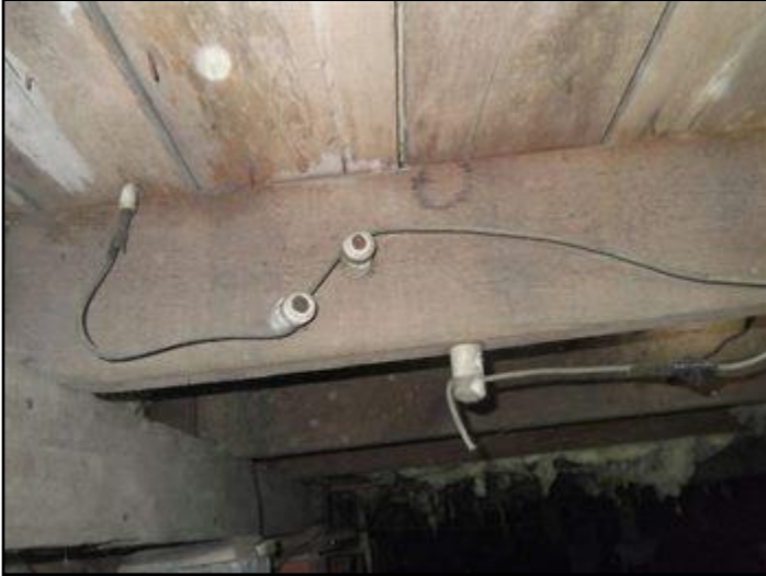
23. Copper - knob and tube
