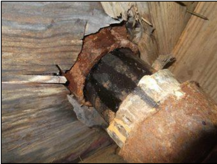
40. Area under toilet showing some leakage.
