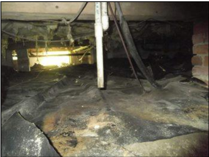
27. Hvac attic unit drains into crawl.
