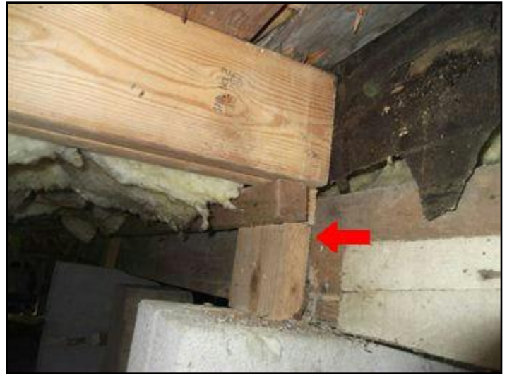
18. Wood joist not supported properly
