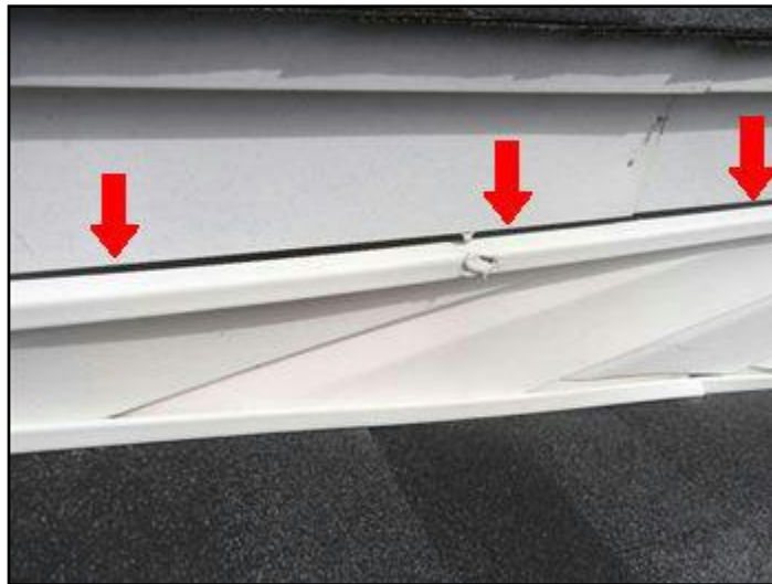
7. Gap between aluminum and vinyl
