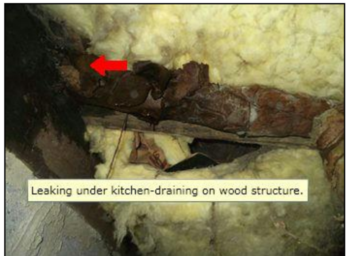
35. Leaking pipe under kitchen
