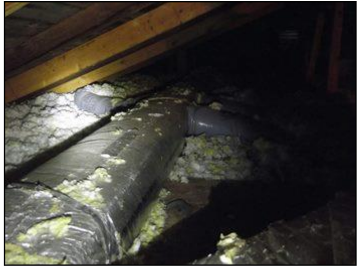
26. Ductwork insulated in attic
