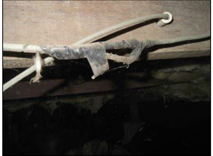
24. Copper - knob and tube
