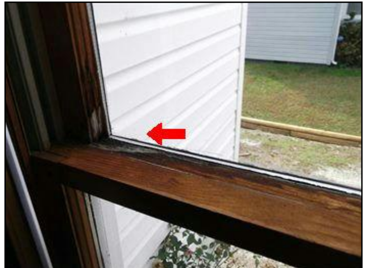
44. Water damage
