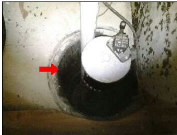
20. Lid missing, rotted or not secure
