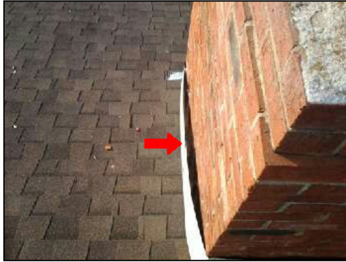
2. Decorative cover flashing not secured...
