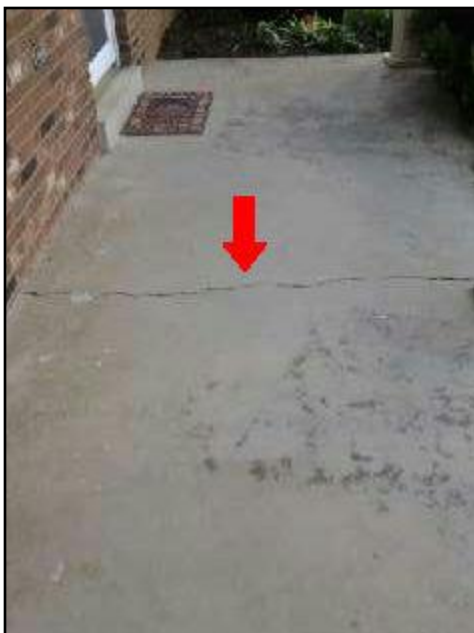
6. Concrete cracked
