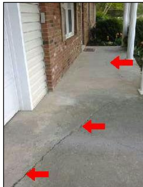
7. Concrete cracked
