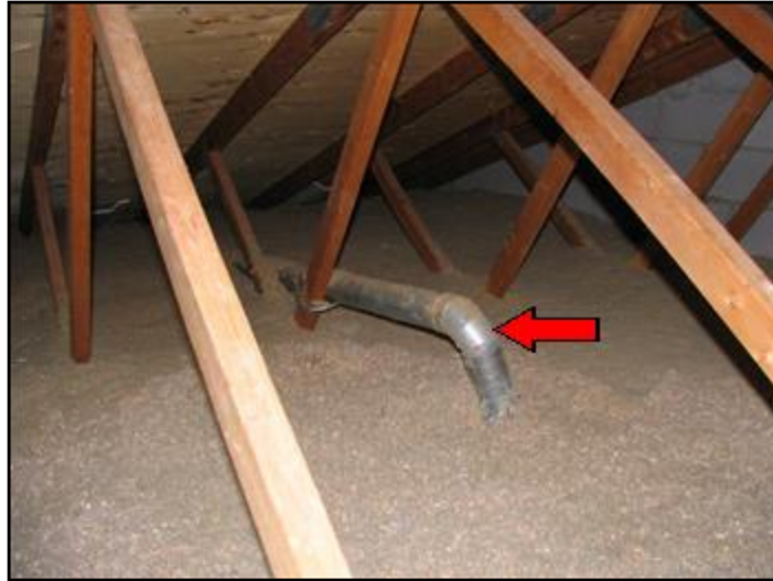
21. Insulate duct work
