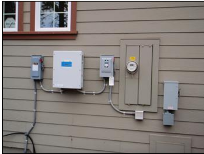
View of solar, main, and generator panel
