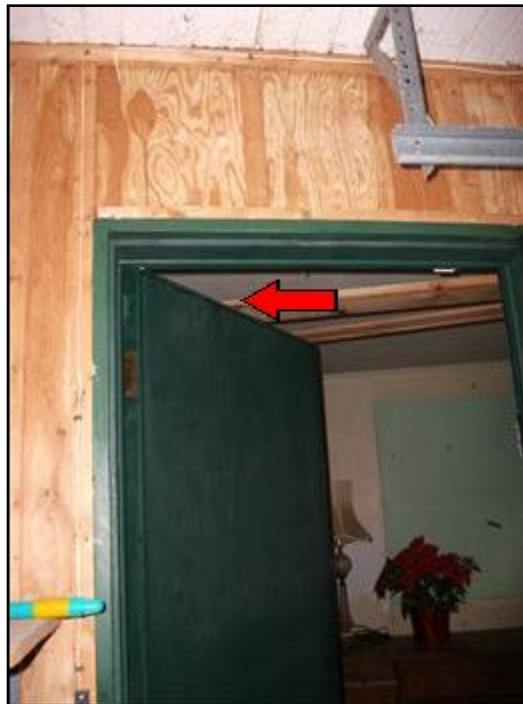
16. Garage Door to House
