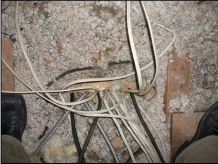
6. Wiring in Attic
