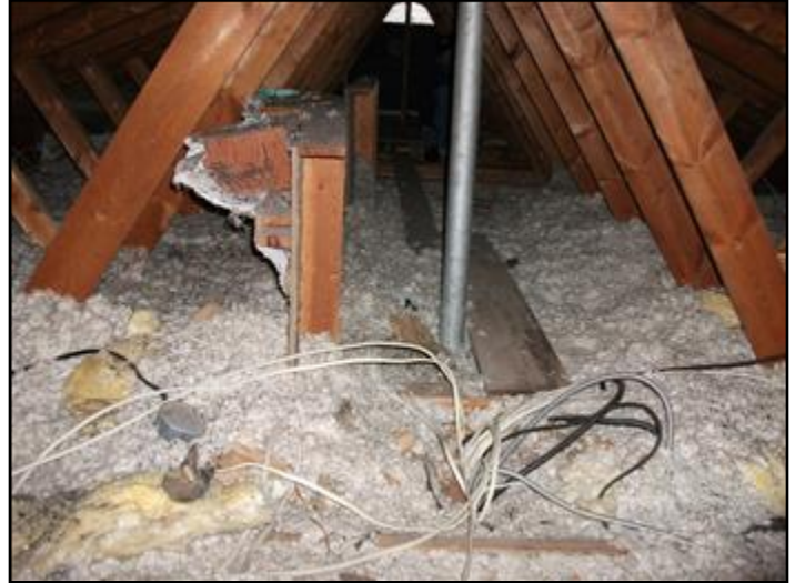
7. Wiring in Attic
