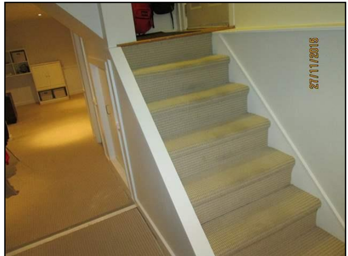
Railing - missing
