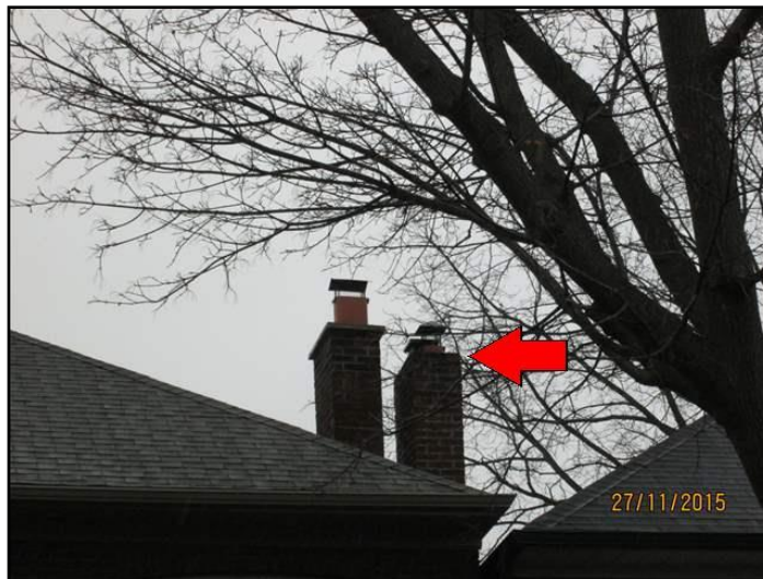
Masonry Cap - missing
