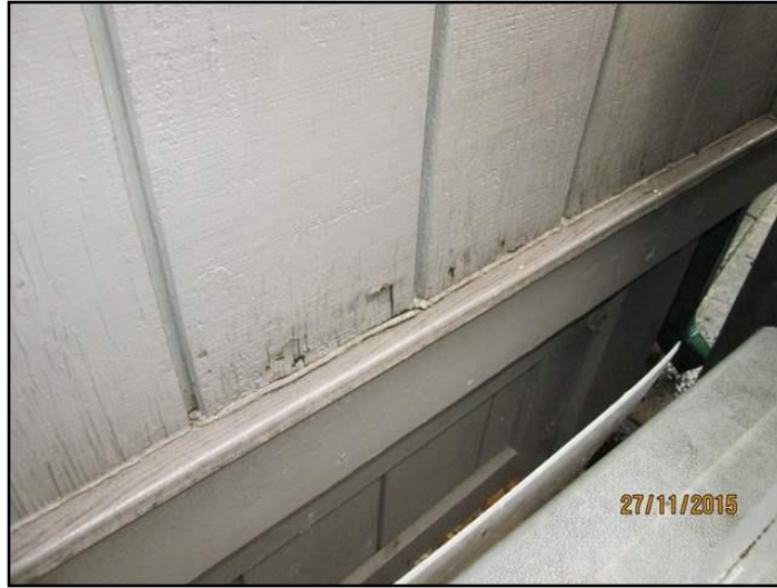
Water damage / rot
