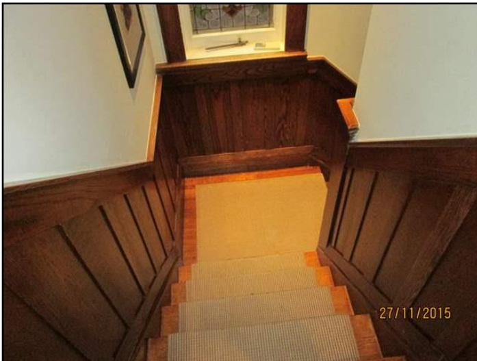
Railing - missing
