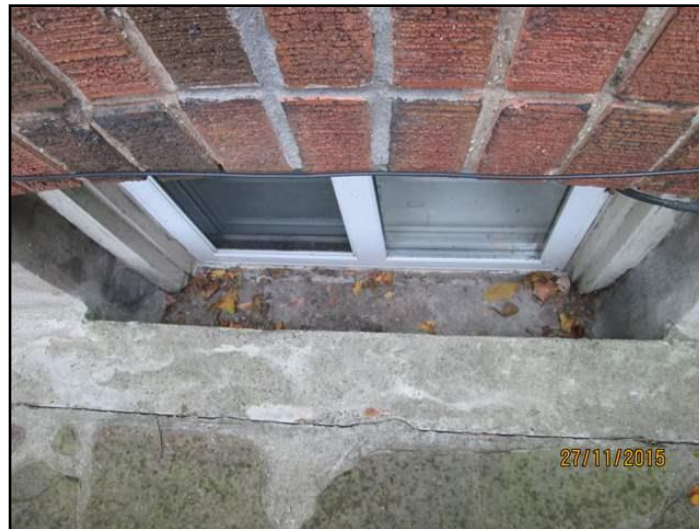
Window Well - missing 6 to 8 inches...
