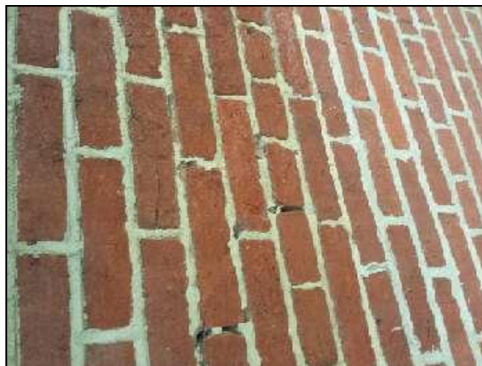
4. Mortar deterioration
