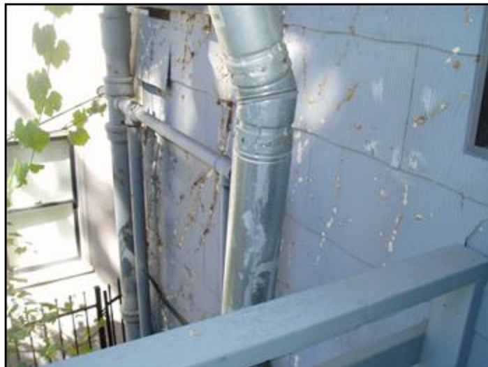
7. THE WATER HEATER FLUE
