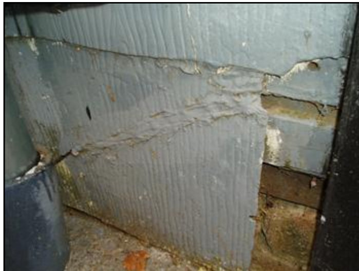
1. CRACKED DAMAGED SHINGLES
