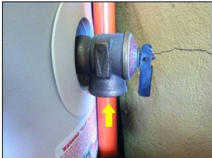
No Discharge Pipe @ TP Valve
