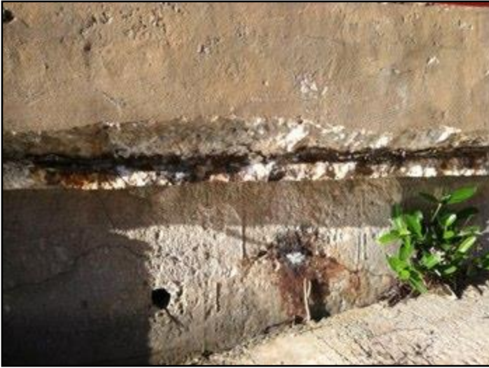
Spalled Concrete
