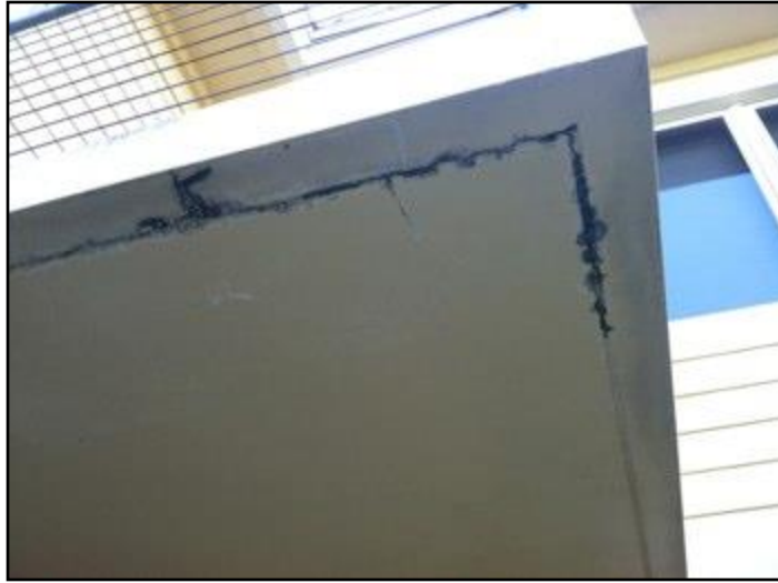
Moisture In Stucco Under Deck
