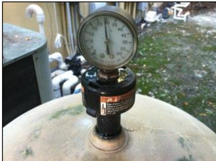
Leaking Pressure Gauge
