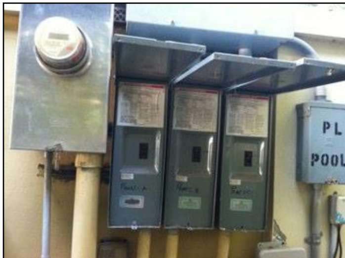
Electric Meter & Disconnects
