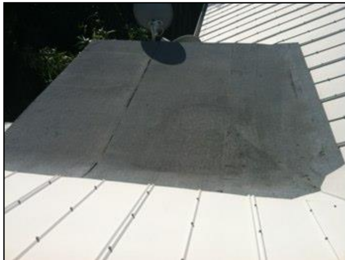
Built-up Roof Over Elevator
