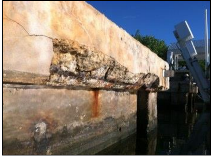
Spalled Concrete
