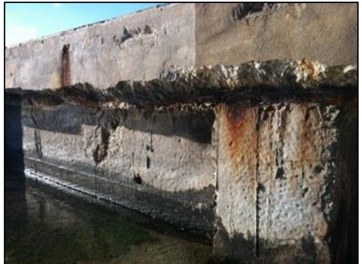
Spalled Concrete
