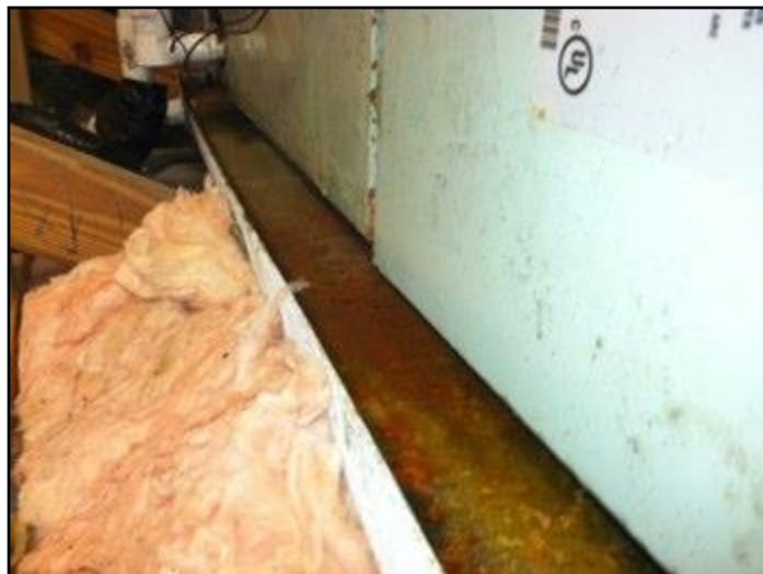
Clogged Condensate Drain(s)
