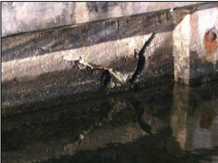
Spalled Concrete
