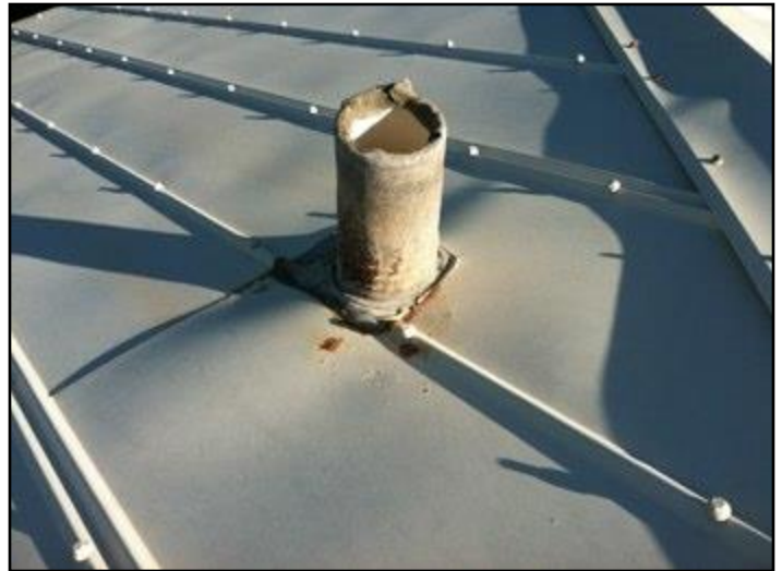
Rusted Roof Panels
