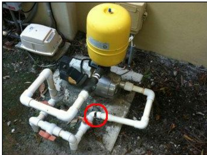
Broken Pressure Tank System
