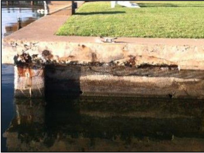
Spalled Concrete
