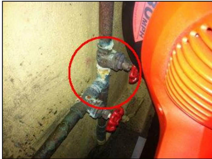
Corroded Pipes
