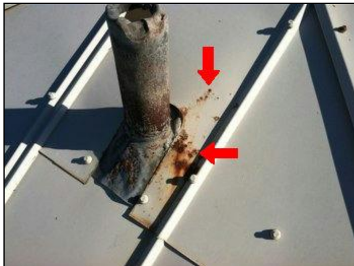
Rusted Roof Panels
