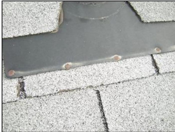
3. Exposed fasteners
