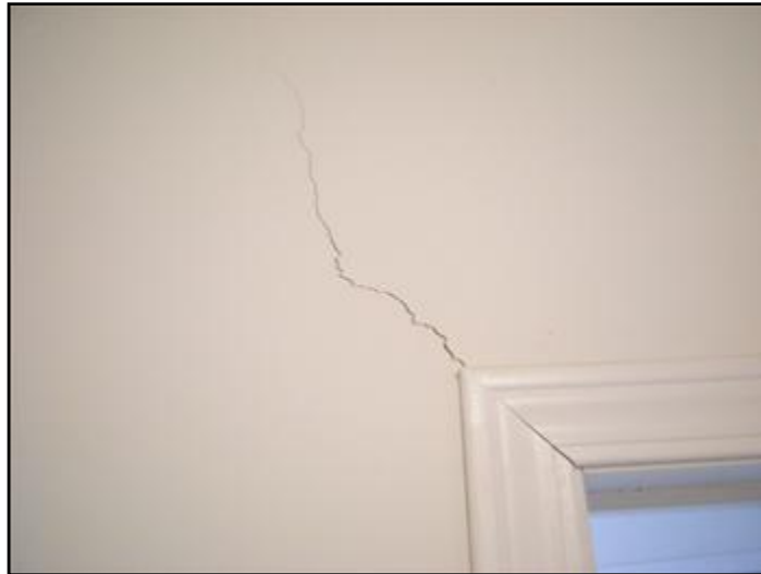
43. Cracked plaster.
