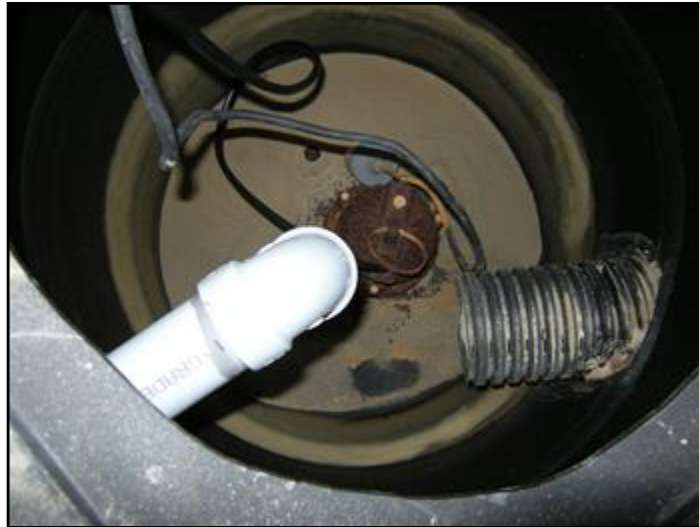
31. Sump basin was dry at time of inspection.
