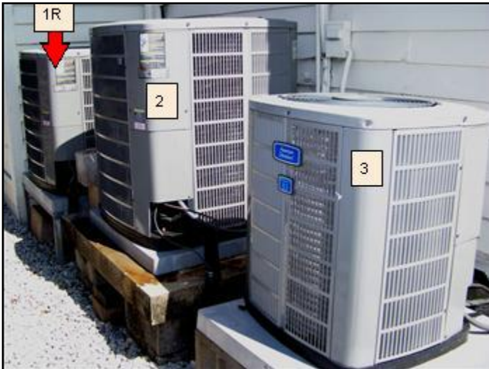
26. AC condensing units 1-3
