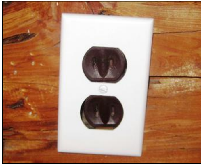
18. Two slotted outlet (ungrounded) 3rd floor
