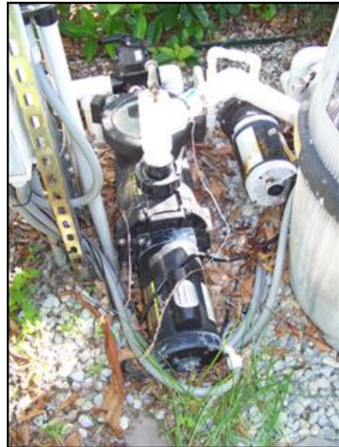
44. Pool pump and motors
