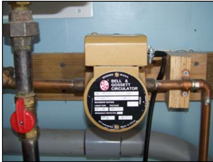
31. Hot water circulating pump
