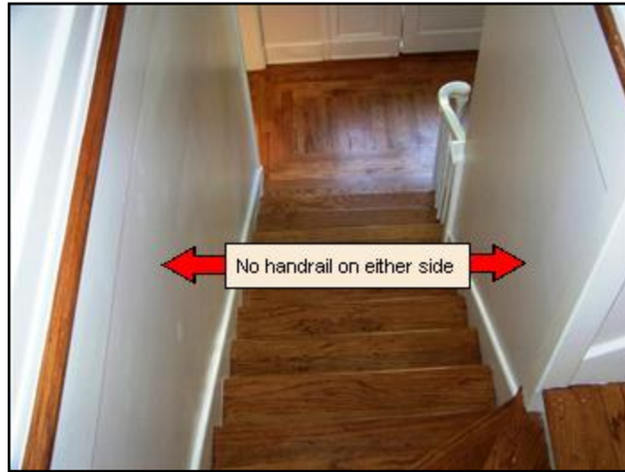
36. Handrail missing - between 1st and 2nd floor
