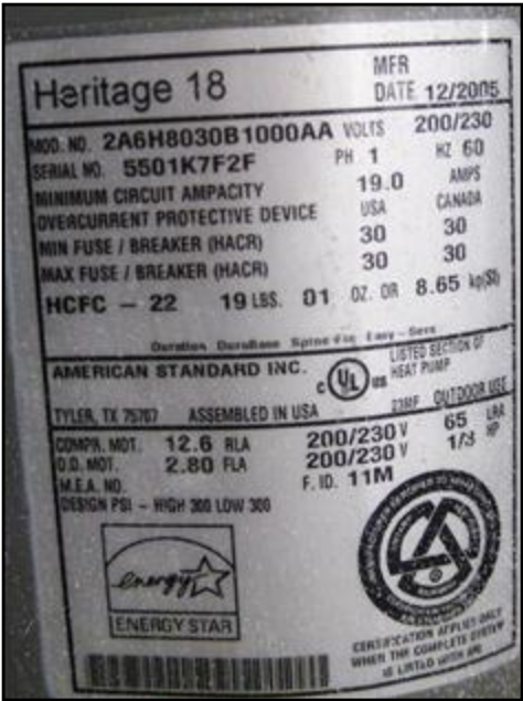
58. AC condensing unit data plate
