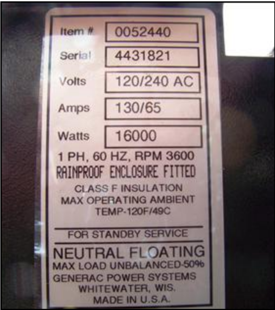
55. Back up generator data plate
