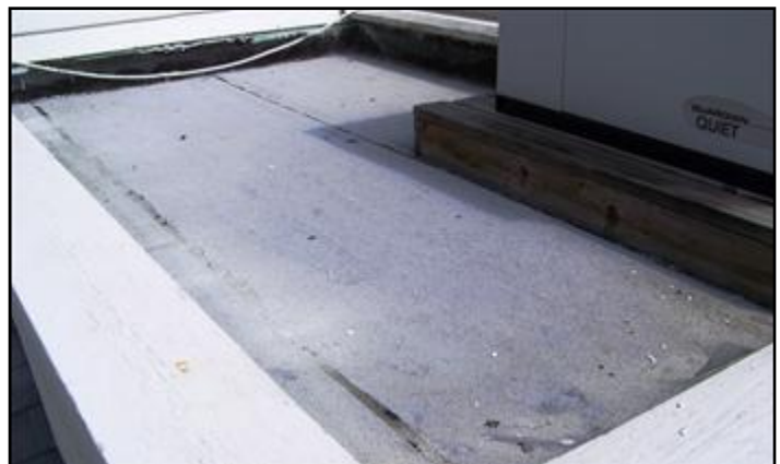
2. Flat roof platform - modified bitumen
