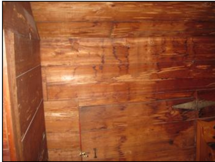
34. Third floor water stains (typical)
