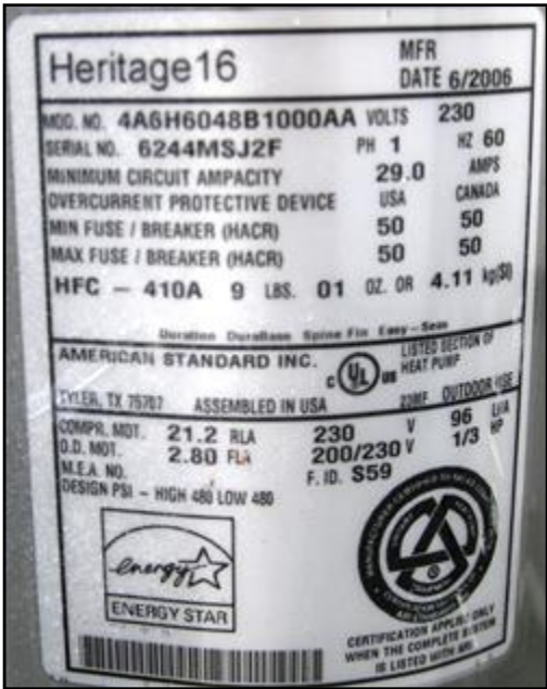
60. AC condensing unit data plate
