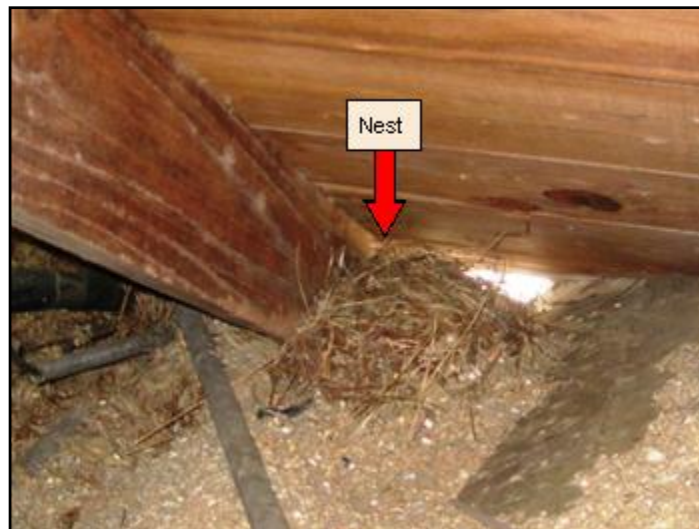
6. Animal or bird nest in attic - open soffit
