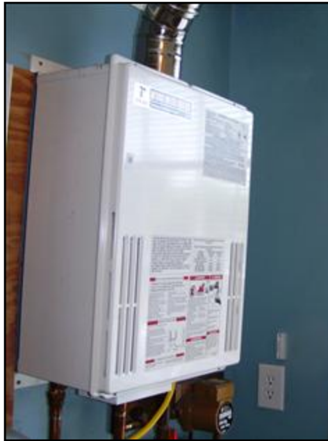
30. Takagi T-M1 tankless water heater
