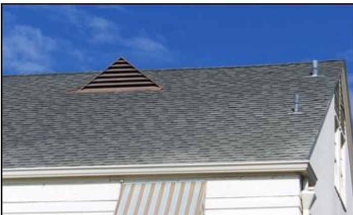
1. Architectural asphalt shingle roof
