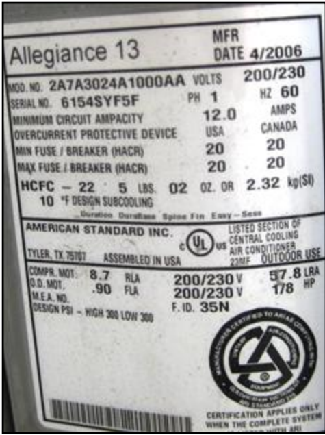
59. AC condensing unit data plate
