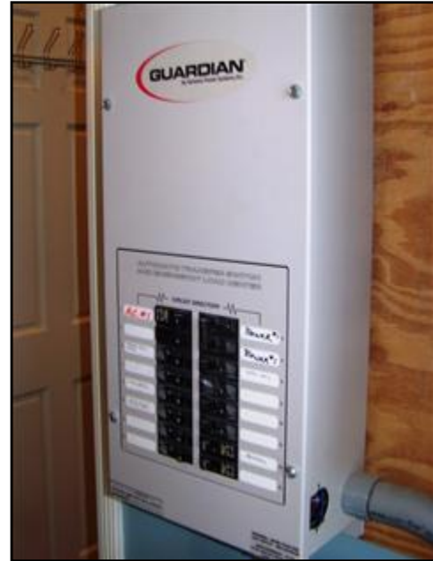
12. Back up generator transfer switch & breakers
