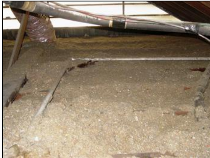
28. Attic insulation (typical) - cellulose
