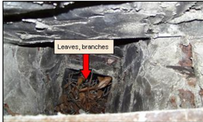
25. 2nd floor fireplace chimney - debris
