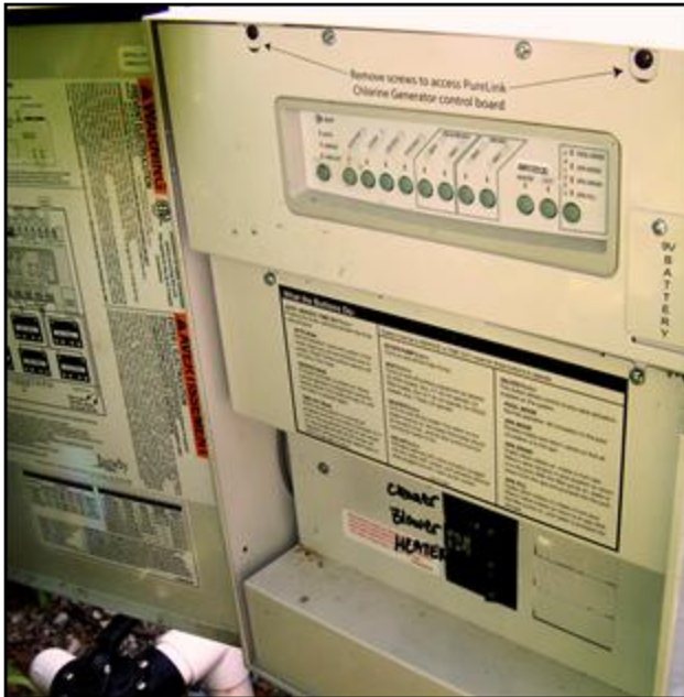
43. Pool control and electrical panel
