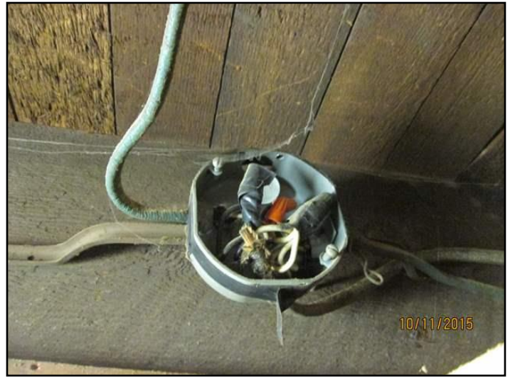
Cover Plate(s) - missing
