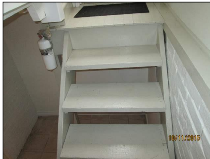
Railing - missing
