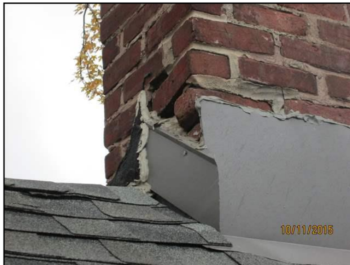
Mortar - deteriorated/missing
