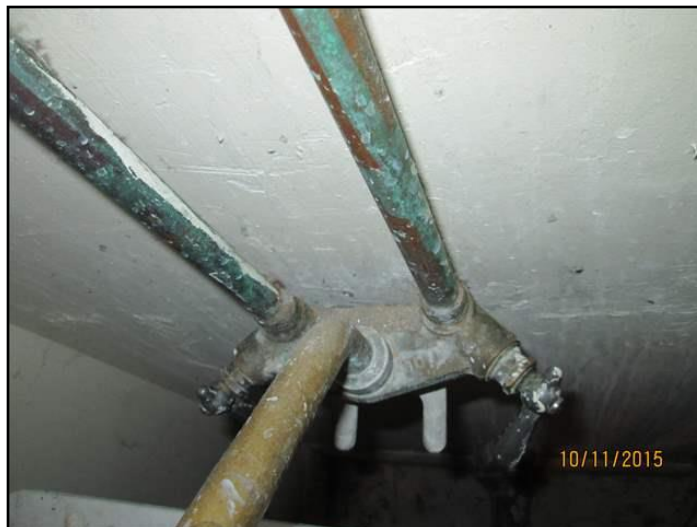
Support inadequate
