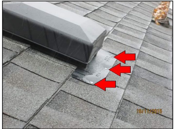
Nail Heads - exposed (risk of leak)
