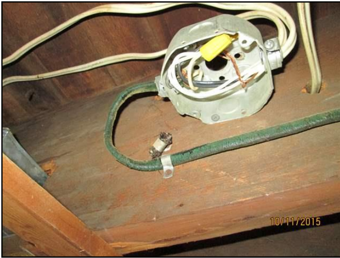
Cover Plate(s) - missing
