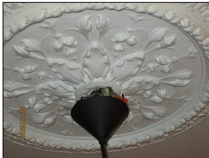
Exposed wiring
