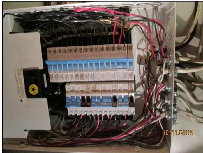
Main panel with cover removed
