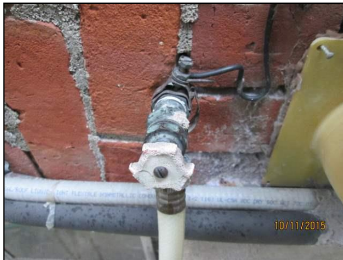
Handle - damage / missing
