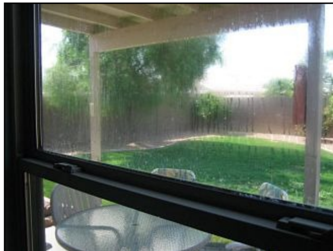
30. Lost seal on double or triple glazing
