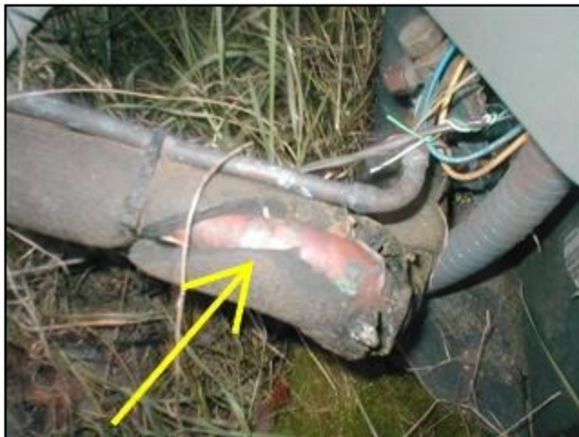
23. Missing insulation
