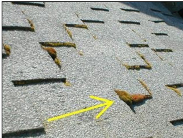
1. Moss/algae growth noted on roof surface. As...
