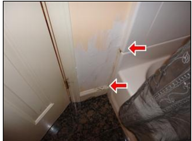
28. Caulking loose, missing or deteriorated
