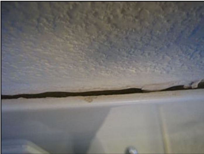
27. Caulking loose, missing or deteriorated
