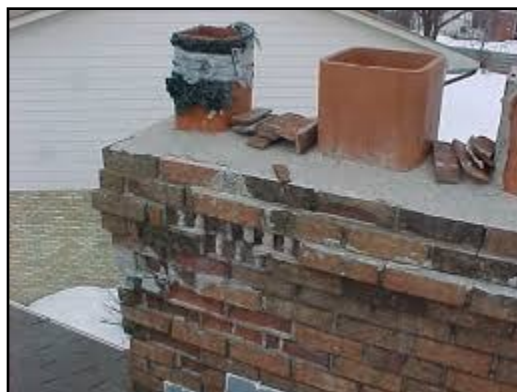
22. Loose, missing or deteriorated masonry
