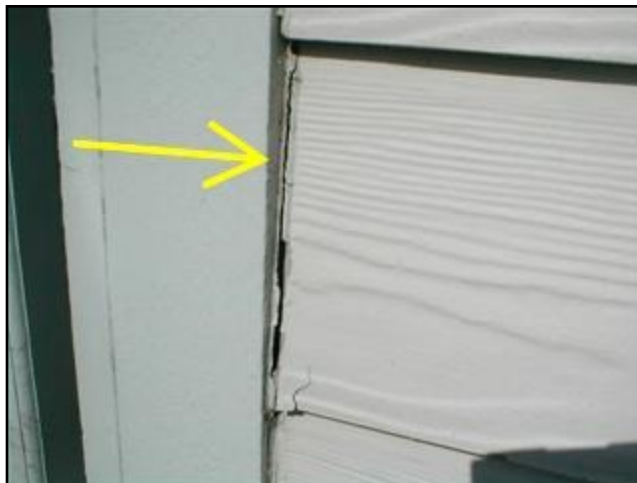
5. Caulking missing or deteriorated
