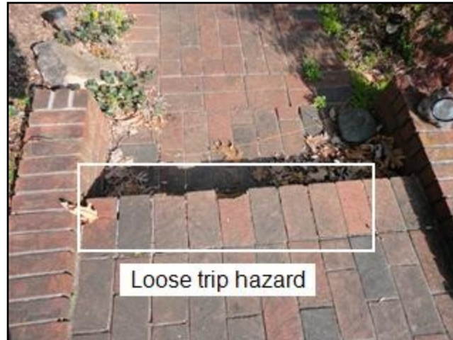
11. Cracked or damaged surfaces
