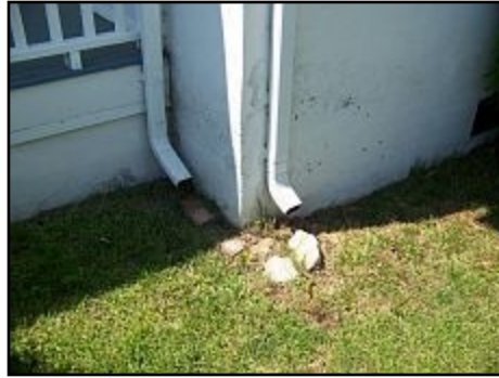
4. Downspouts end too close to building
