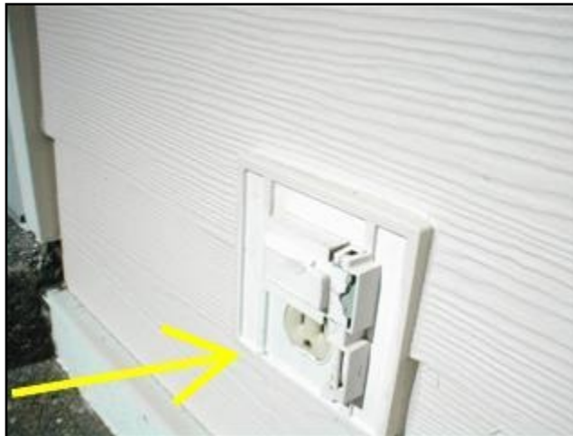
18. No GFI (Ground Fault Interrupter)
