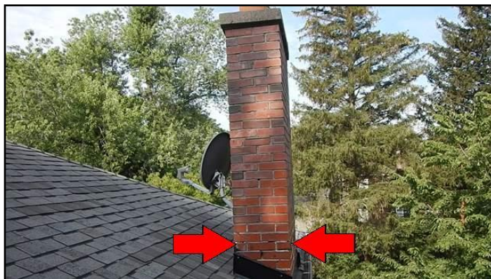
Mortar - deteriorated/missing
