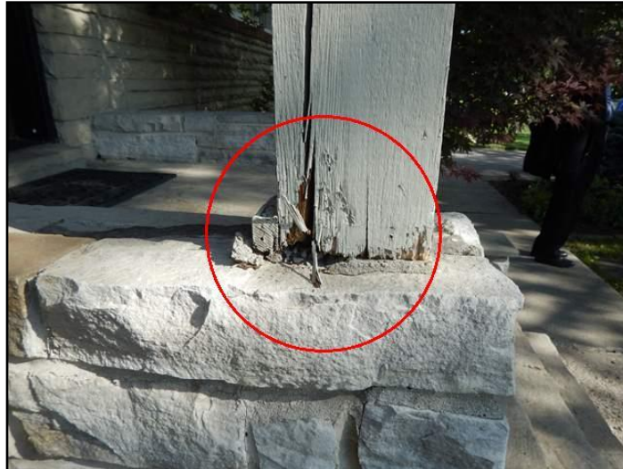
Water damage / rot
