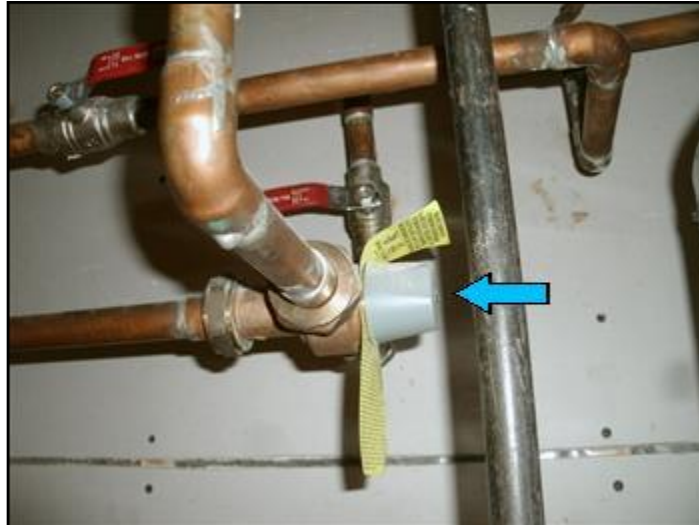
Tempering (mixing) Valve noted
