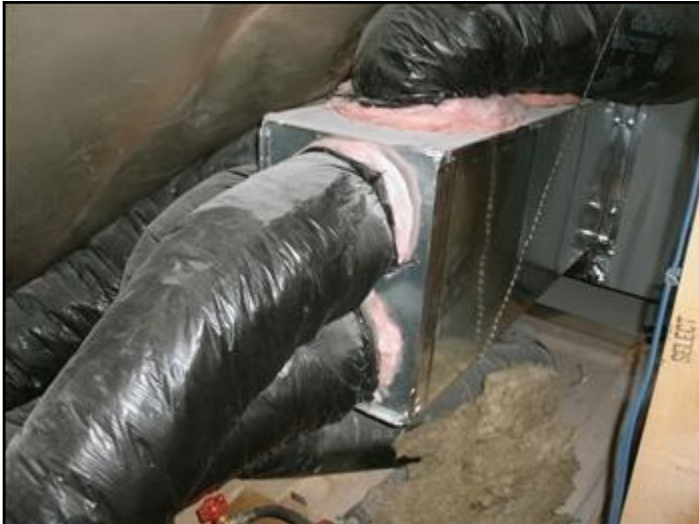
Air handler in 3rd floor knee wall.
