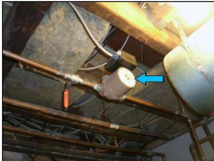
Circulating loop in place
