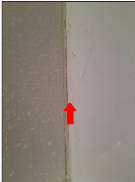
Caulking loose, missing or deteriorated
