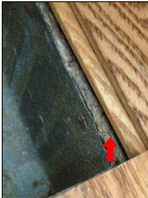
Possible asbestos insulation around heating...
