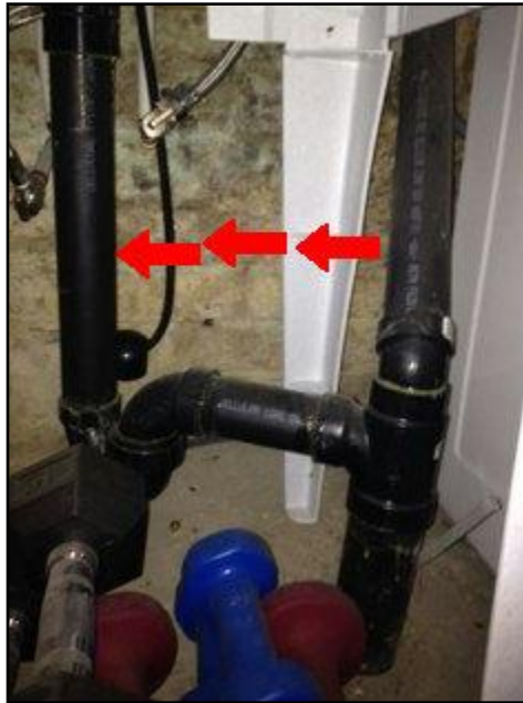
Drain on wrong side of trap
