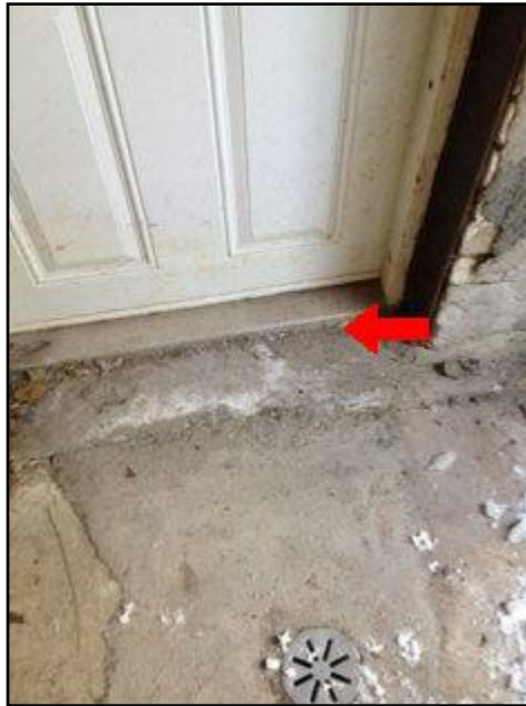
Door threshold missing, too low, not...
