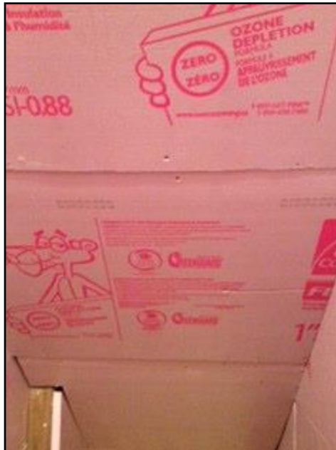
Exposed combustibile insulation
