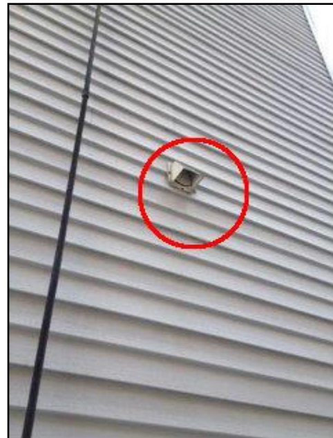
Caulking missing or deteriorated
