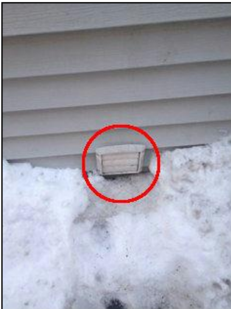
Caulking missing or deteriorated
