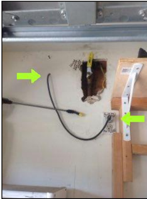
26. Extension cord used as permanent wiring
