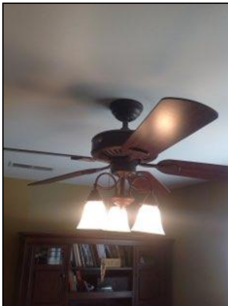
27. Light functioned but fan did not
