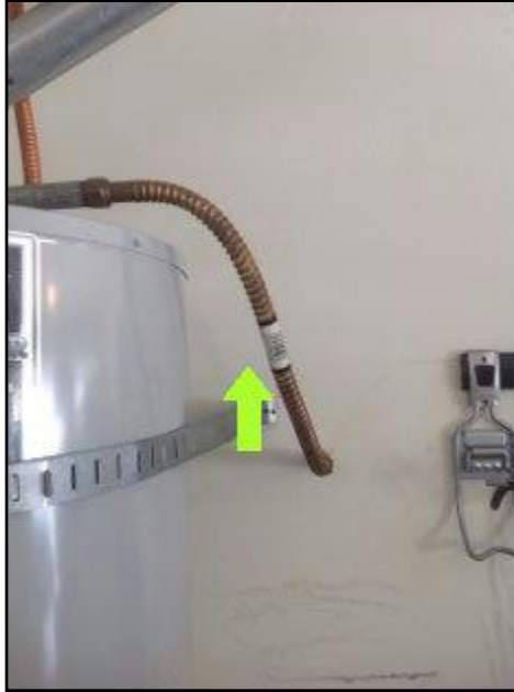
11. Improper material used for TPR discharge pipe
