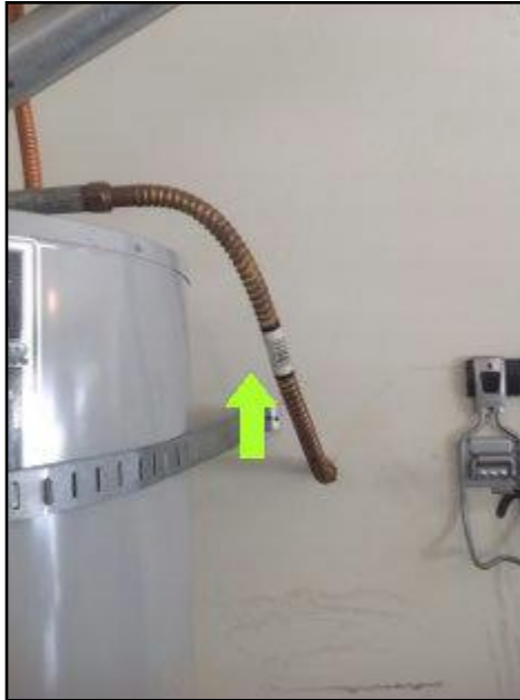
37. Improper material used for TPR discharge pipe
