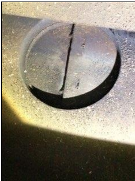
31. Damper in existing fireplace not fixed open
