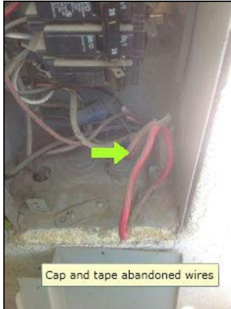
25. Abandoned wires in panel
