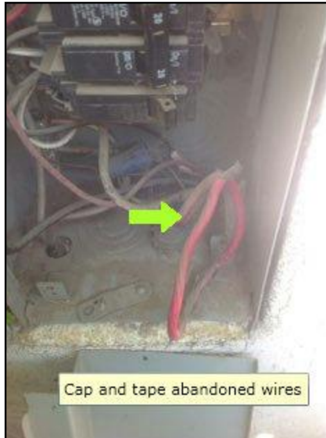
5. Abandoned wires in panel
