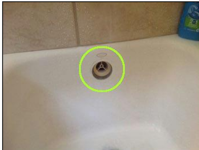
41. Overflow cap missing
