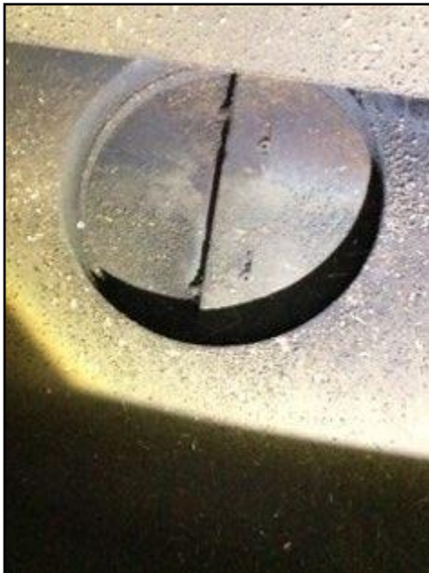
9. Damper in existing fireplace not fixed open
