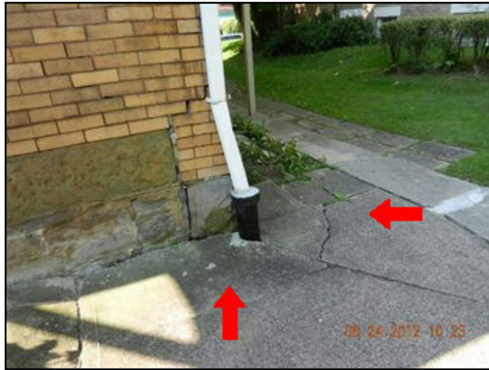
8. Improper slope or drainage
