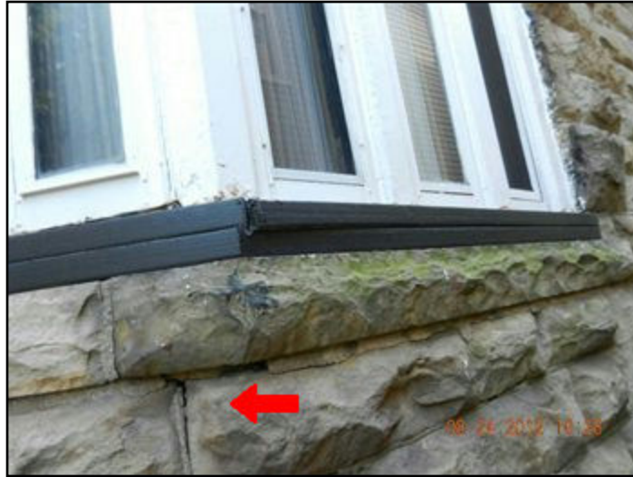
7. Mortar deterioration
