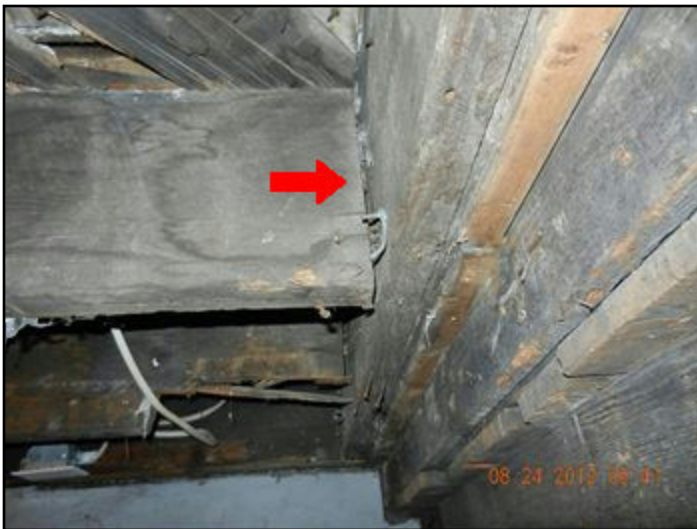
10. Poor end bearing, joist hanger connections
