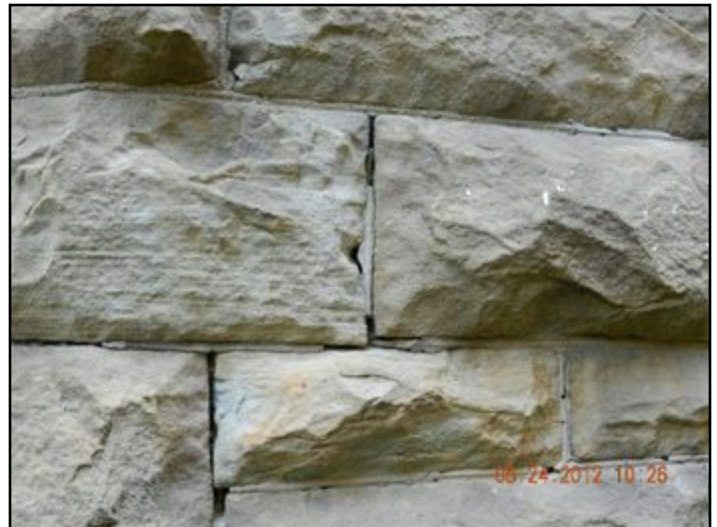
6. Mortar deterioration
