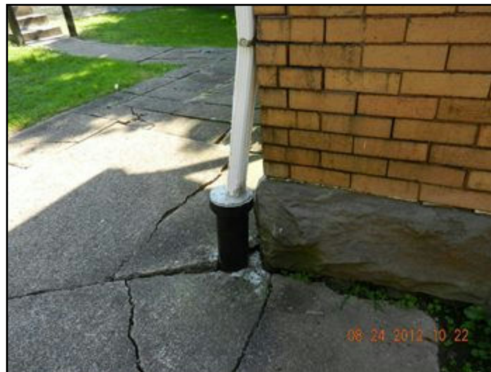
4. Downspouts discharging below grade
