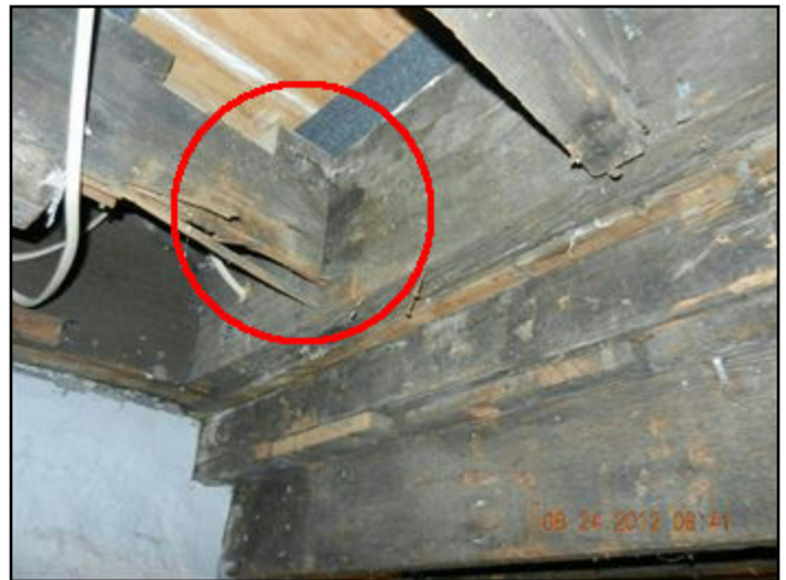
11. Poor end bearing, joist hanger connections
