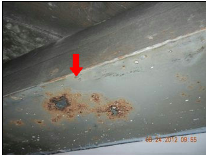
20. Rusted HVAC return duct
