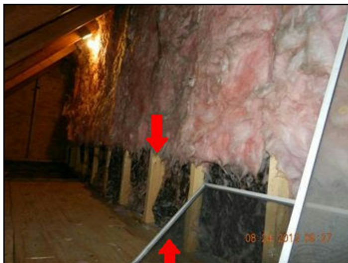
25. Inadequate in knee wall areas
