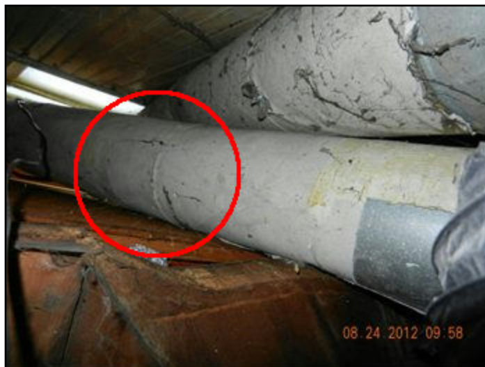
21. Asbestos lining ductwork
