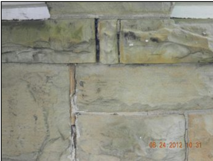
5. Mortar deterioration
