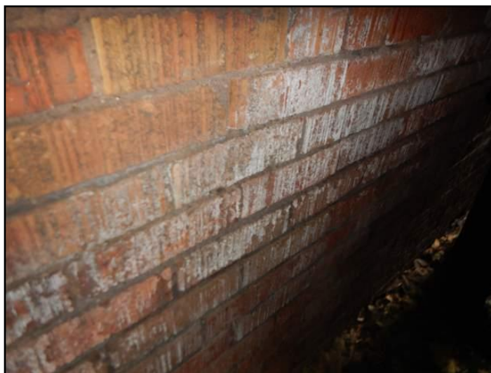
Example - Efflorescence
