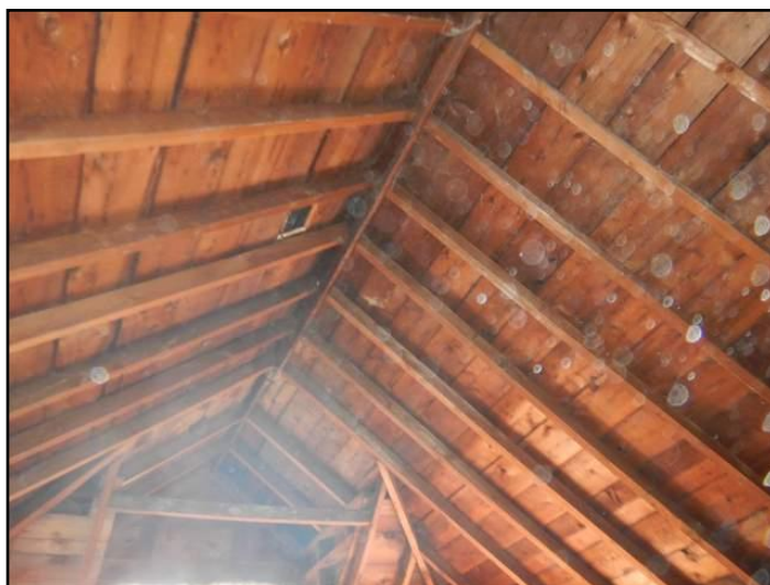
Rafters/ceiling joists
