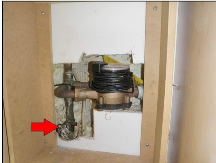
Front of the basement
