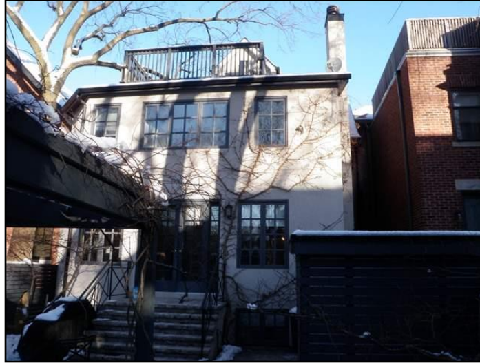
Vines may damage the home -
