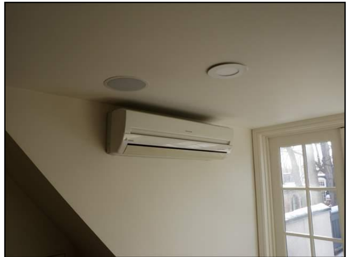
Ductless (Mini split) system- indoor unit
