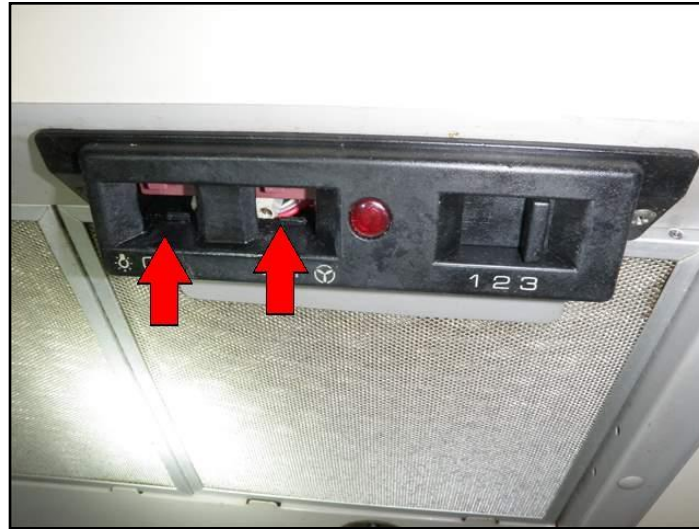
Missing sliders at fan and light switches
