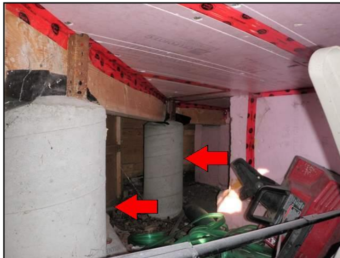
Piers at rear portion of addition
