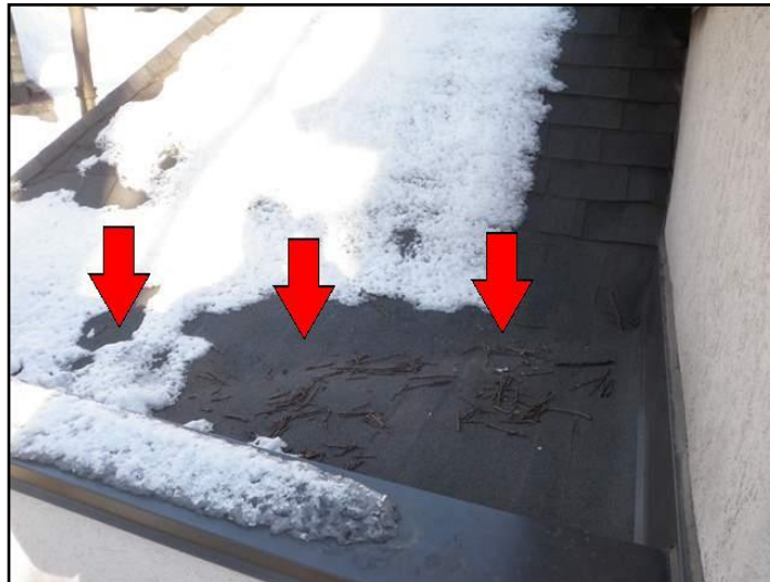
Modified bitumen membrane in runoff area
