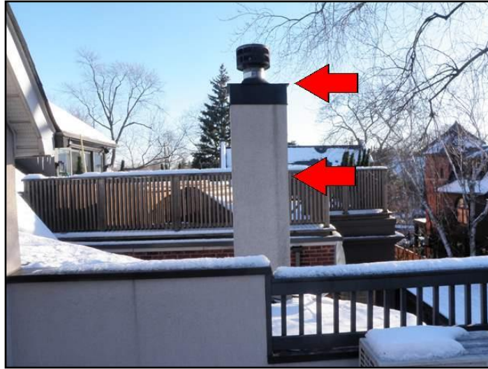
Stucco over metal
