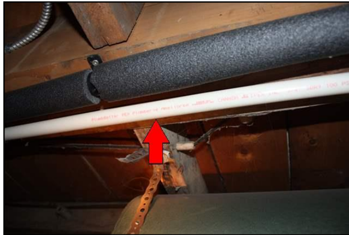
15. IPEX piping (Kitec, PlumbBetter, IPEX AQUA,...)
