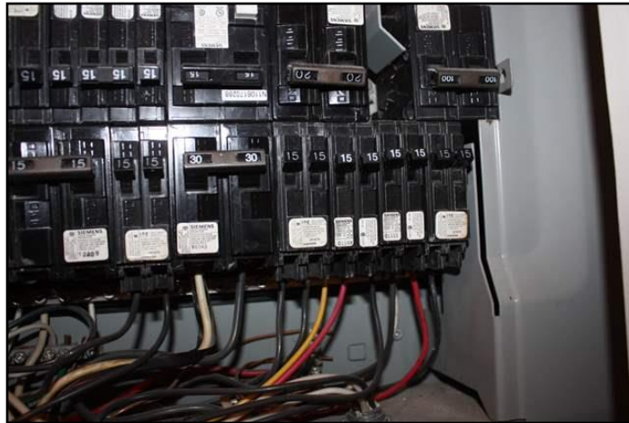
9. No links for multi-wire circuits
