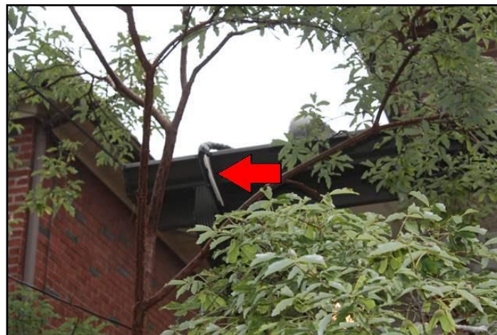
12. Insulation - missing
