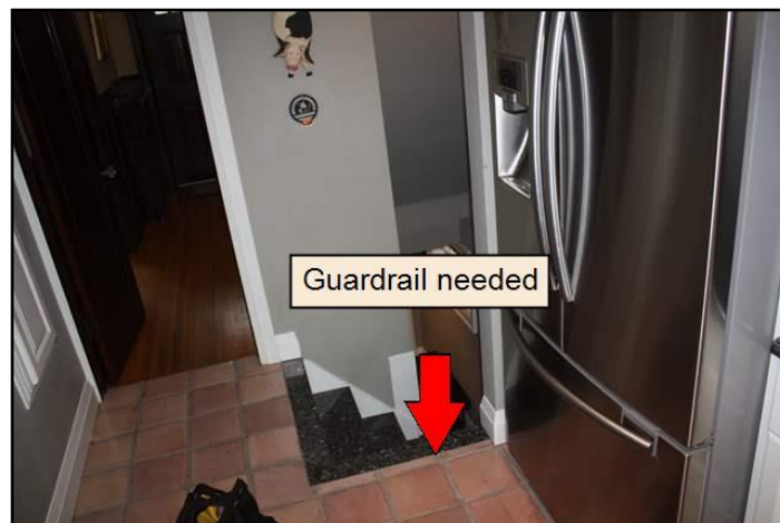
18. Missing Guardrail
