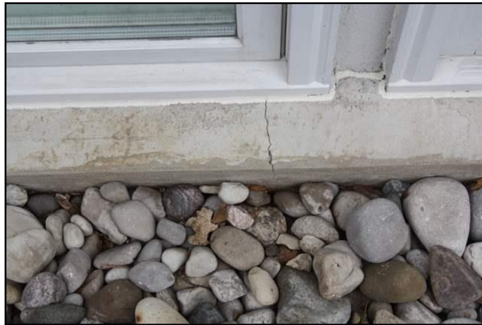
7. Typical minor cracks
