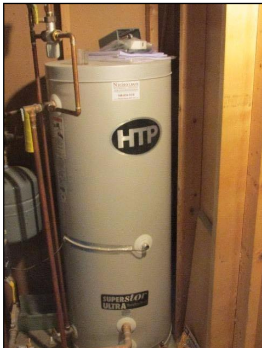
33. SuperStor Indirect hot water storage tank...
