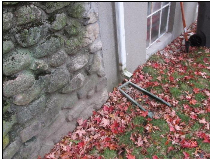
15. Should discharge 6 feet from building
