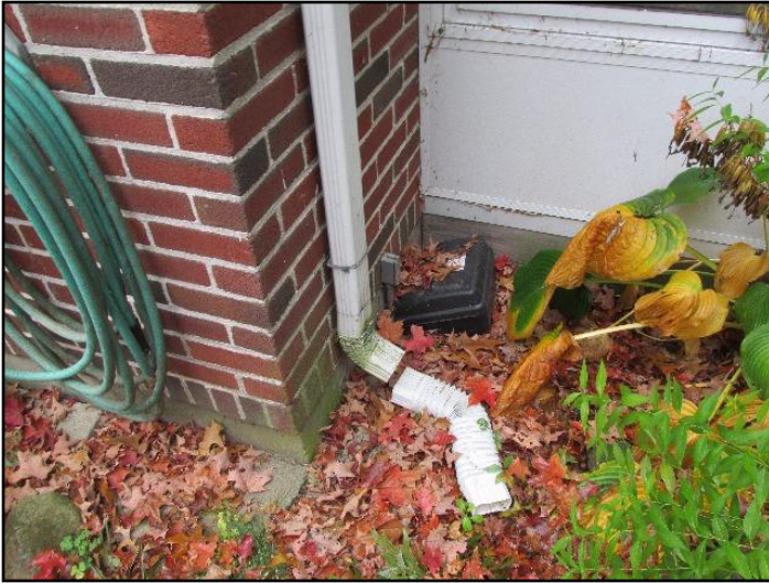
13. Not connected to leader/not extended
