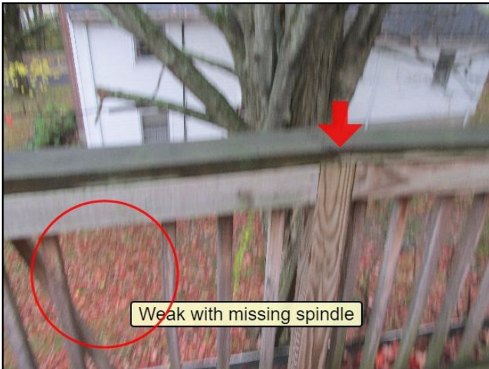
25. Rot or insect damage
