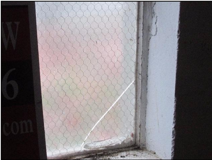
16. Caulking missing or deteriorated
