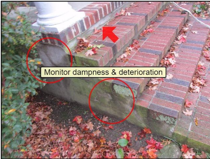
20. Masonry or concrete spalling
