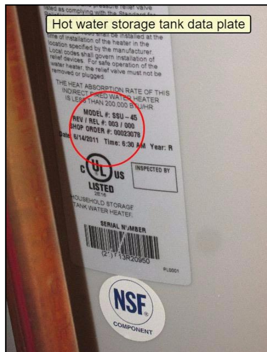
34. SuperStor Indirect hot water storage tank...
