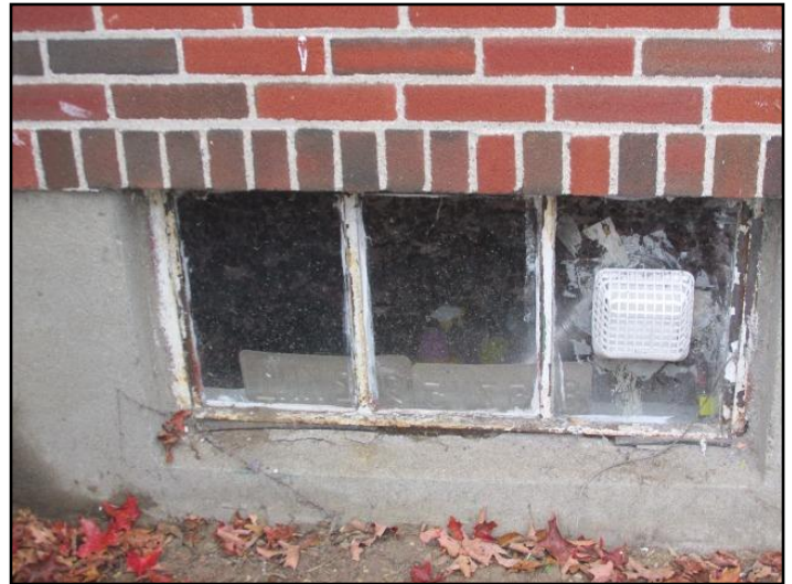
17. Caulking missing or deteriorated
