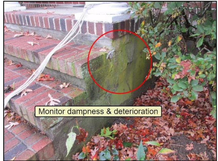
21. Masonry or concrete spalling
