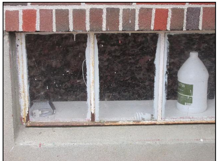
19. Caulking missing or deteriorated
