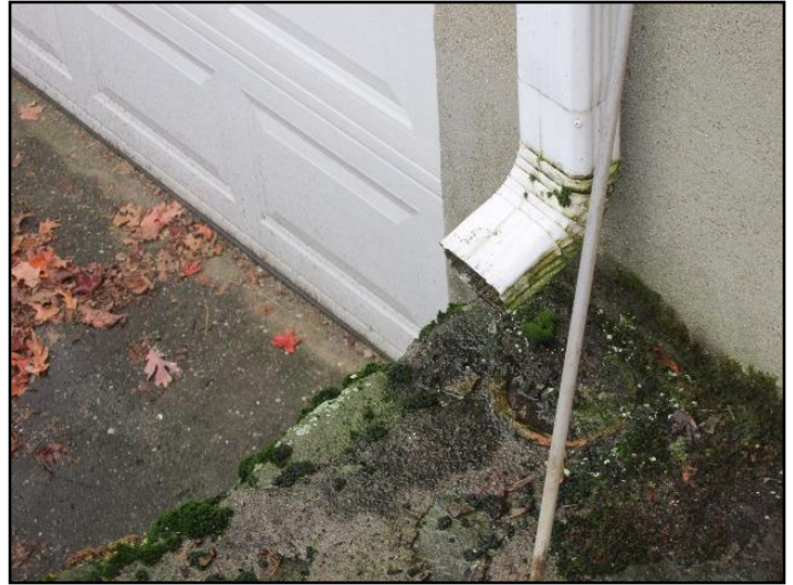
14. Should discharge 6 feet from building
