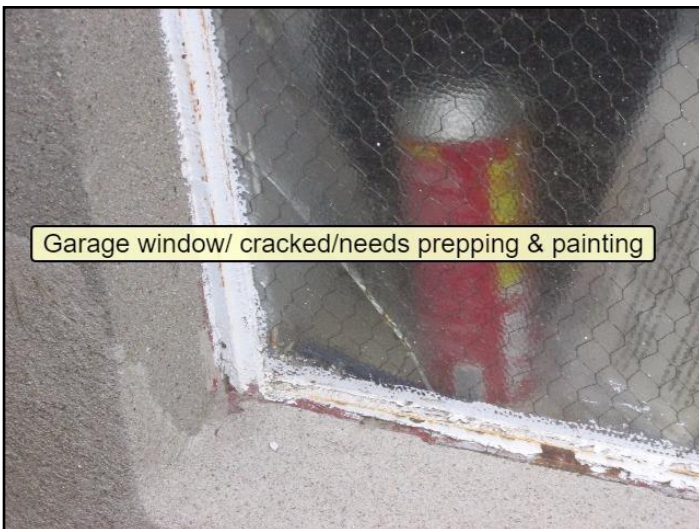
18. Caulking missing or deteriorated
