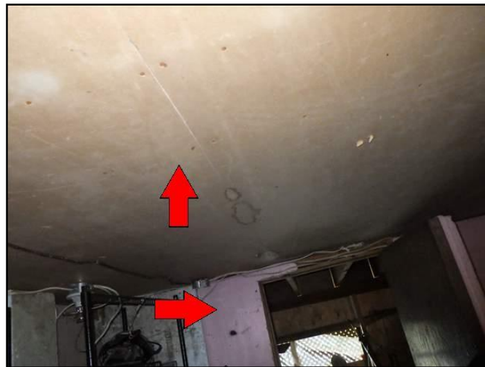
Exposed combustible insulation
