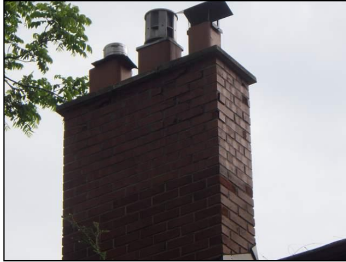
Loose, missing or deteriorated masonry
