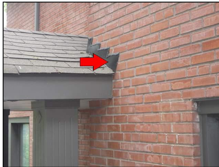
Kickout flashing - missing
