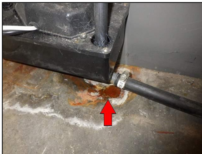
Condensate leak
