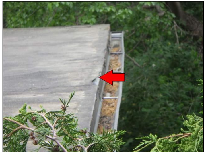
Edges, seams and/or flashings - loose, open
