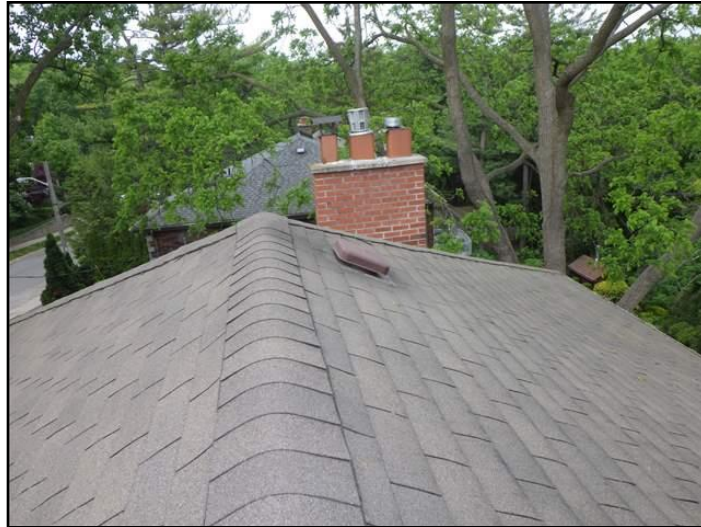
Asphalt shingles
