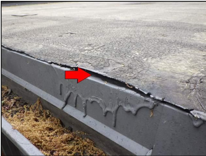
Edges, seams and/or flashings - loose, open
