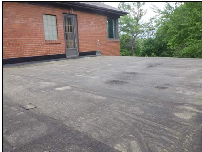
Modified bitumen membrane
