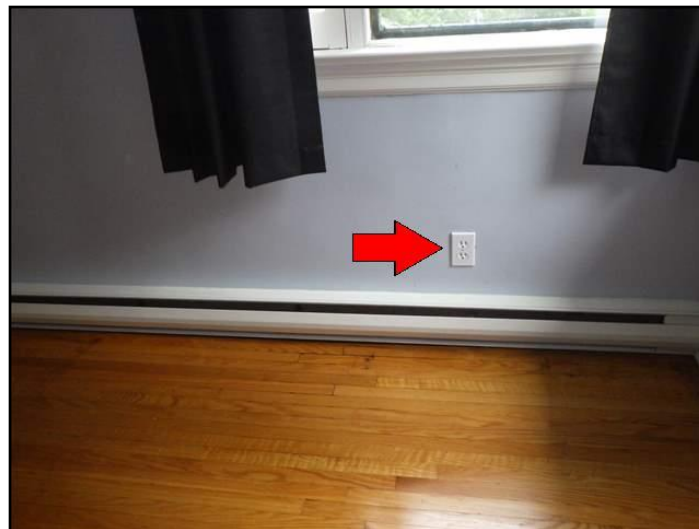
Electrical receptacle above heater
