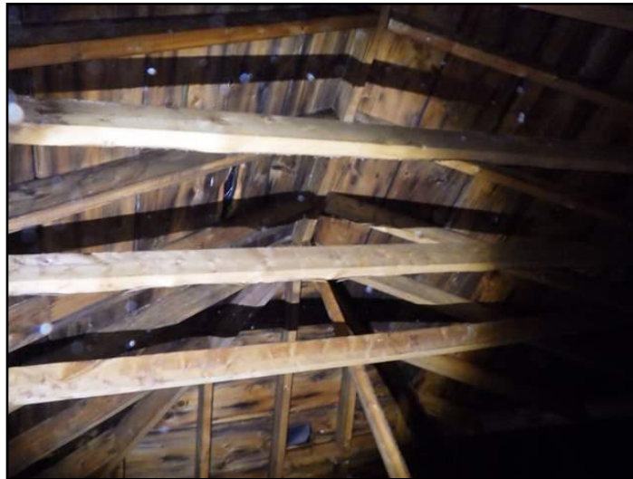
Rafters/ceiling joists
