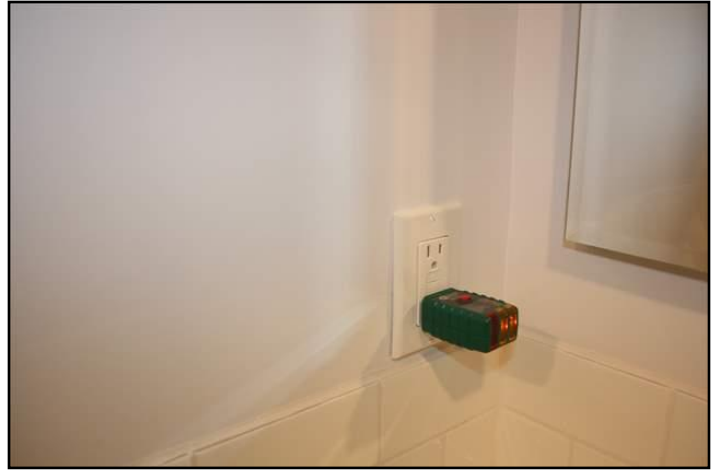
25. Test faulty on GFCI/GFI (Ground Fault...
