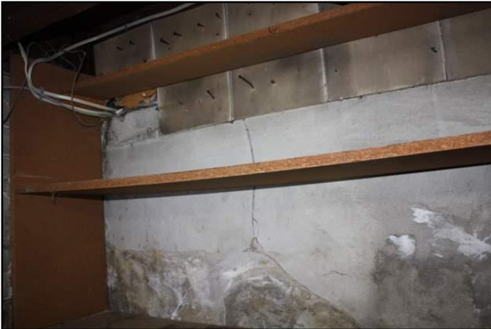
20. Parging damaged or missing
