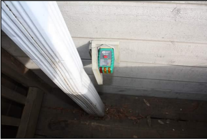
24. Test faulty on GFCI/GFI (Ground Fault...
