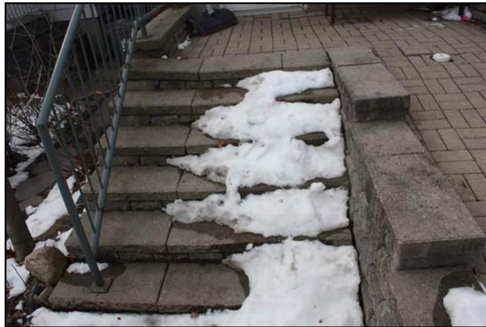
10. Steps or landings settling or heaving
