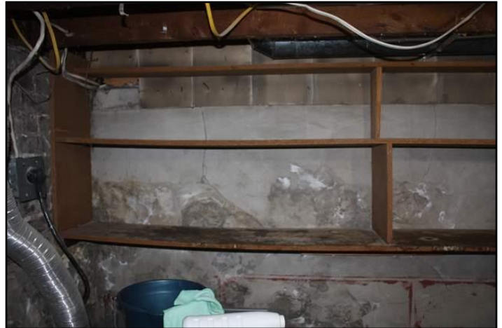
21. Parging damaged or missing
