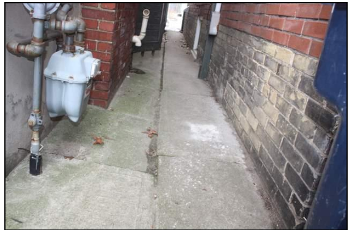
14. Improper slope or drainage
