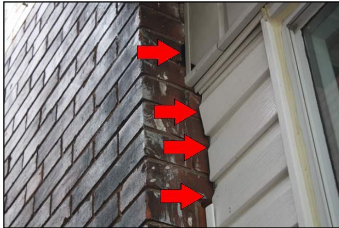
Gaps at wall should be sealed
