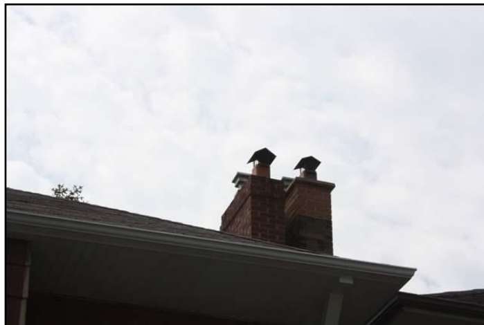
Masonry Cap - missing
