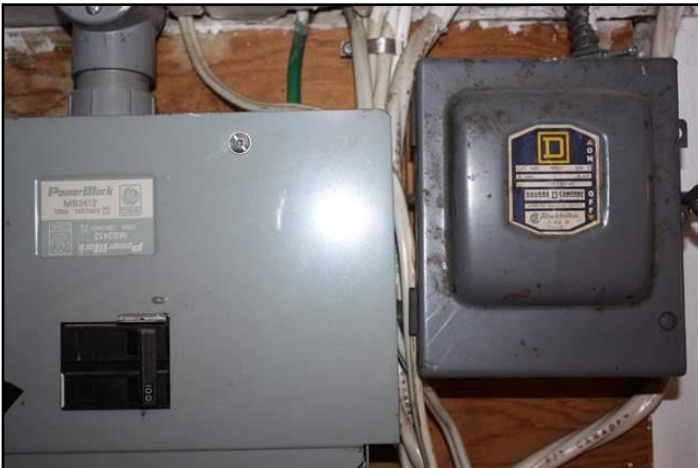
Disconnect missing at Main Panel
