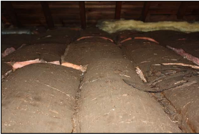
Insulation level below modern standards
