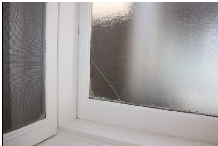
Glass - cracks
