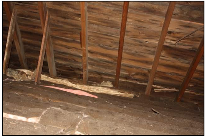
Insulation level below modern standards
