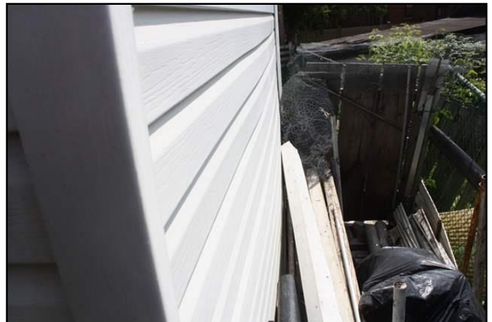
Rear garage wall bowing noted
