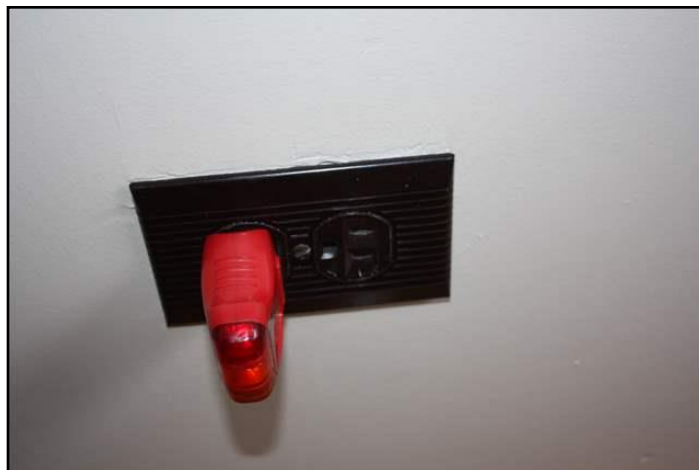
Reversed polarity (black / white wires...)
