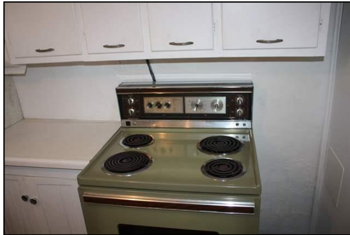
Combustible clearance inadequate
