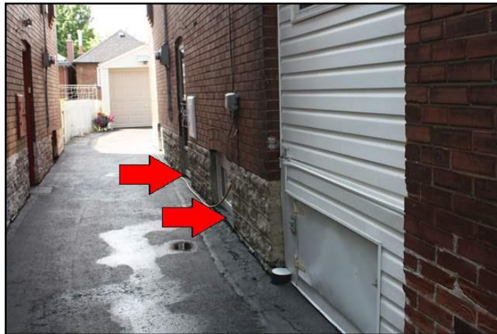
Sill - clearance inadequate (above grade...
