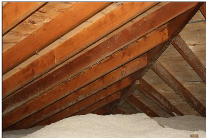
Insulation level below modern standards
