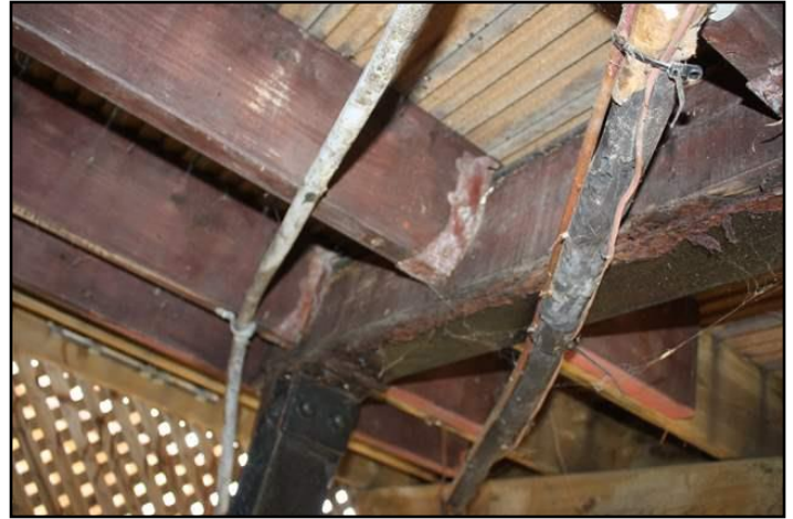
Joist hangers rusted
