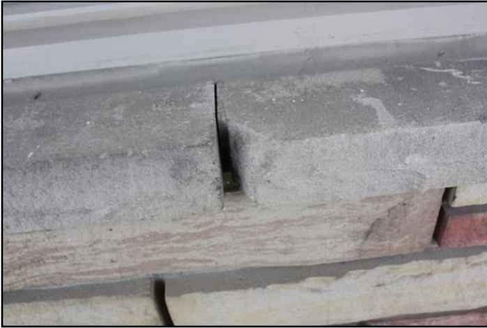
Mortar - missing from sill
