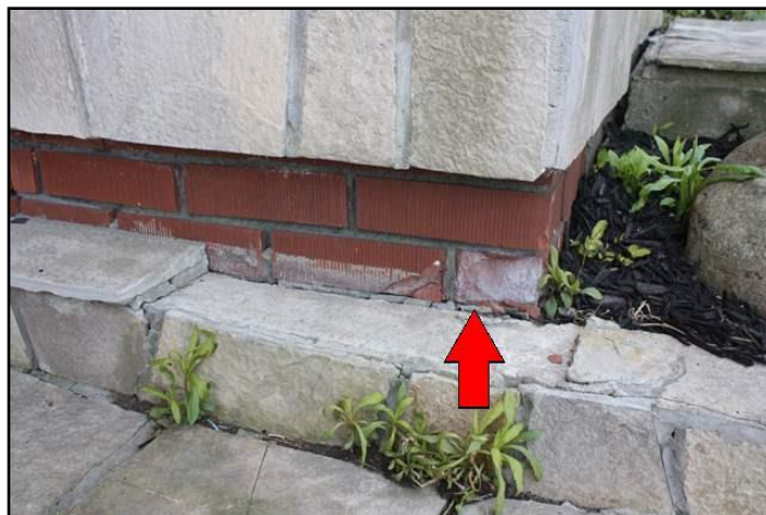
Example Spalling surfaces
