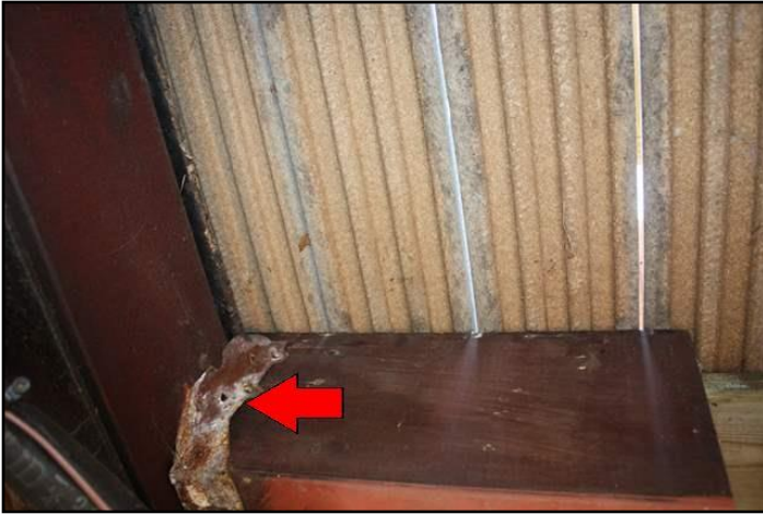
Example joist hangers rusted
