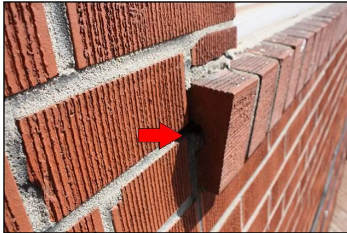
Gap at wall should be sealed
