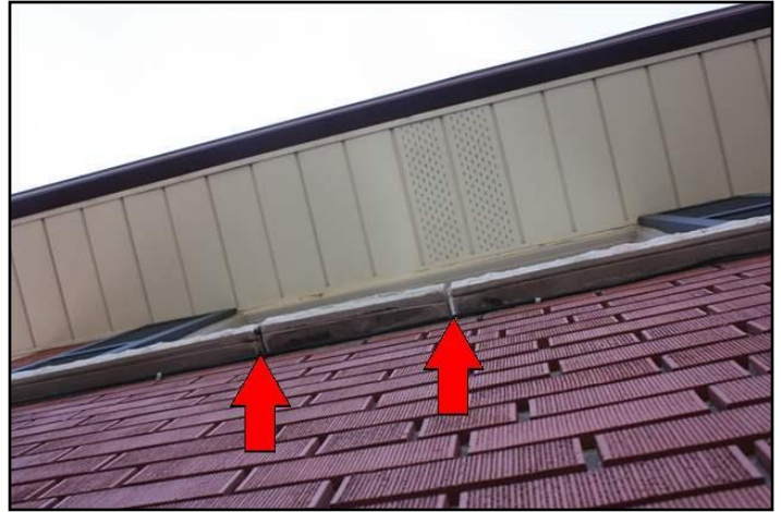
Mortar - missing from sill
