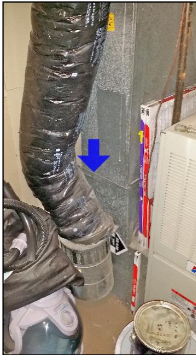
Air Dam Combustion Air
