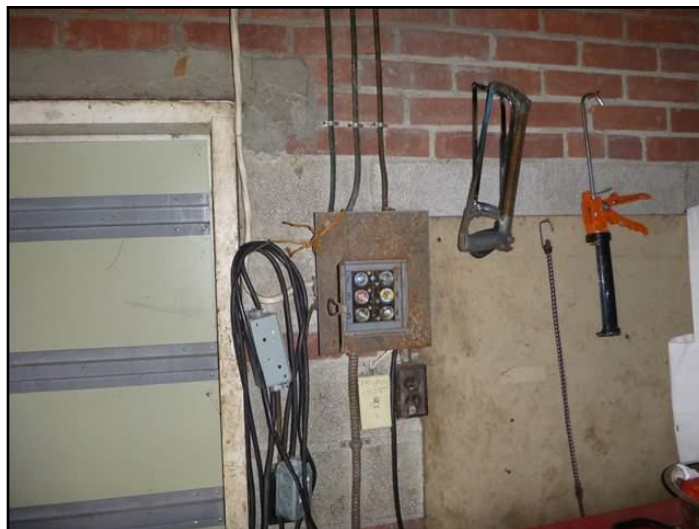
Fuse panel in garage- not in use
