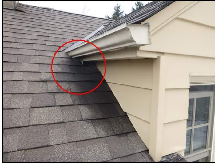
Discharge onto roofs
