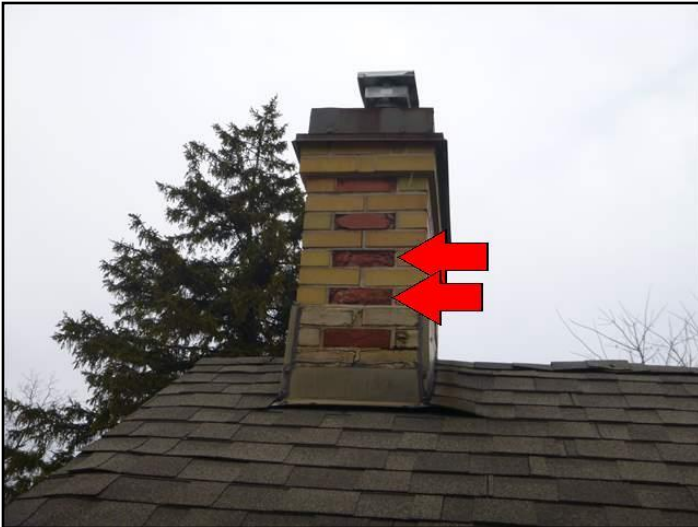
Masonry deterioration noted
