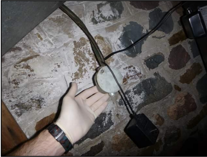
Loose junction box (near panel)
