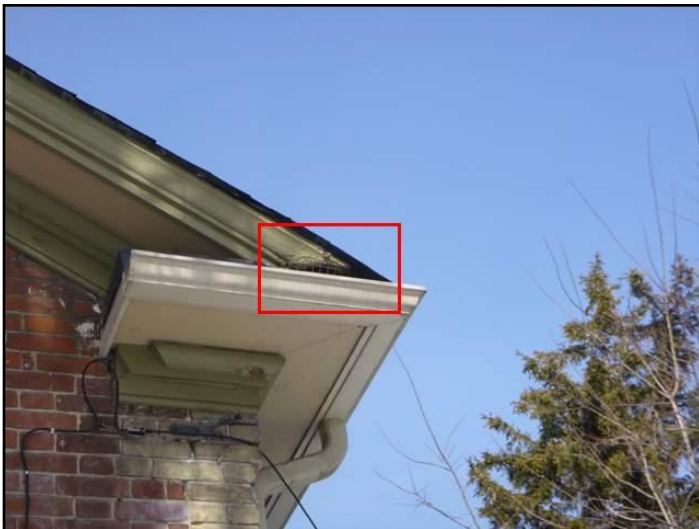
Screens noted at soffit/fascia
