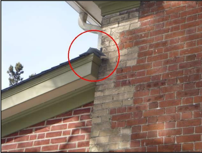
Loose flashing noted
