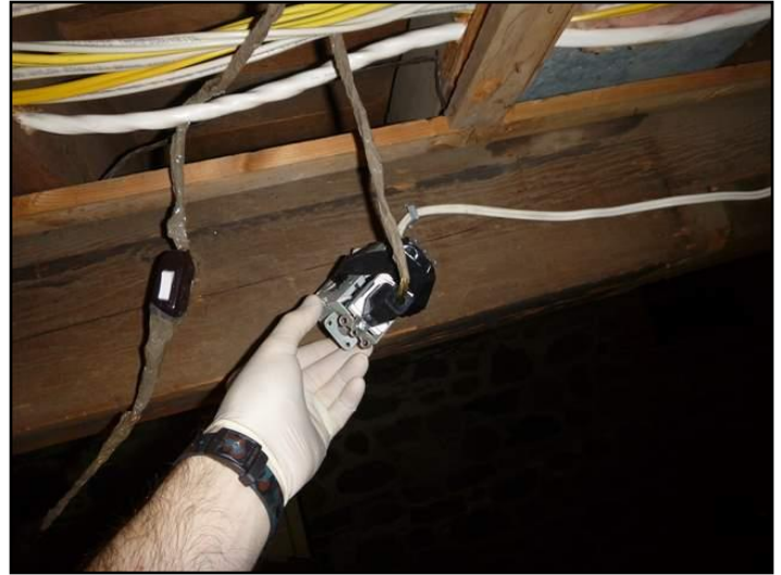
Loose outlet junction box (pool table area)
