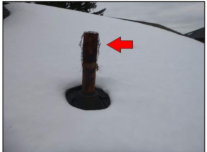
Screens noted at plumbing stack
