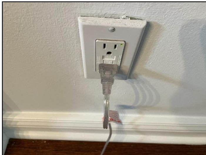
11. example of gfi outlet in ungrounded area
