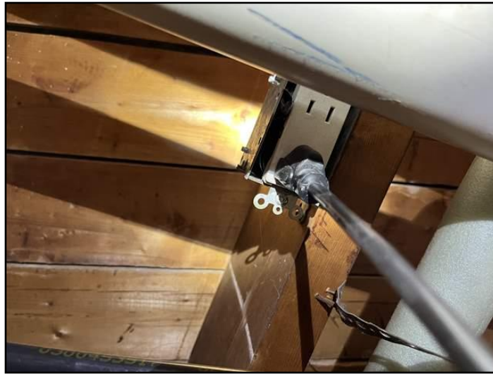
13. For outlet (receptacle) is missing
