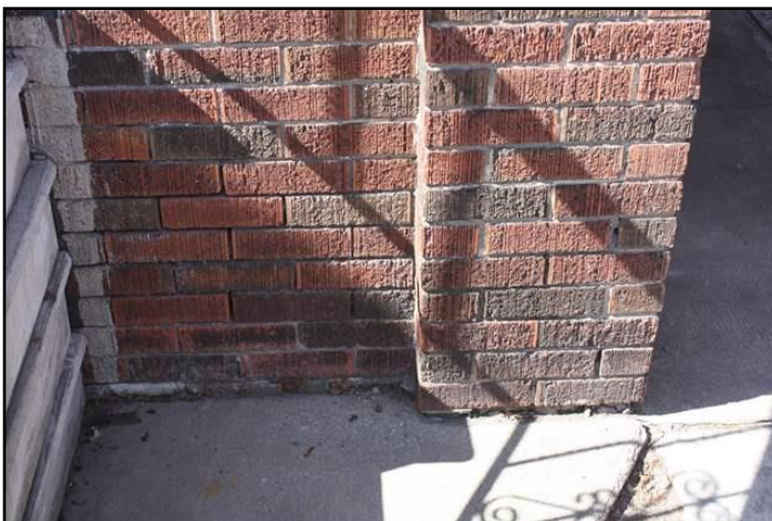
4. Spalling
