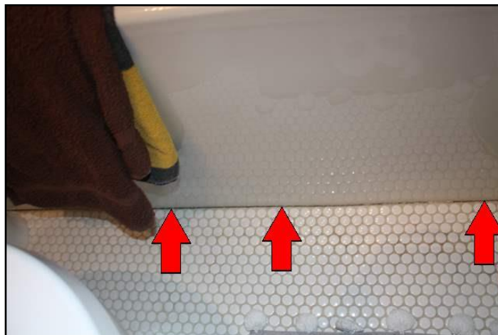
19. Caulking loose, missing or deteriorated
