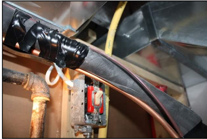
14. For switch is missing
