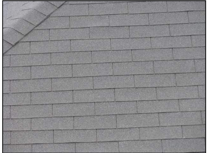
Asphalt shingles
