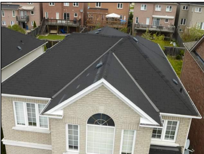
Asphalt shingles - front
