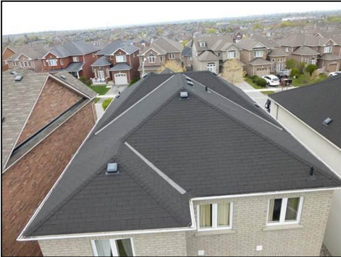
Asphalt shingles - rear
