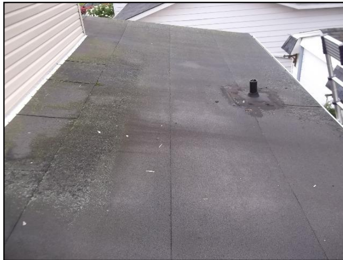
10. Modified bitumen
