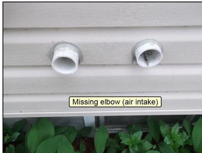
71. Outside - sealed combustion
