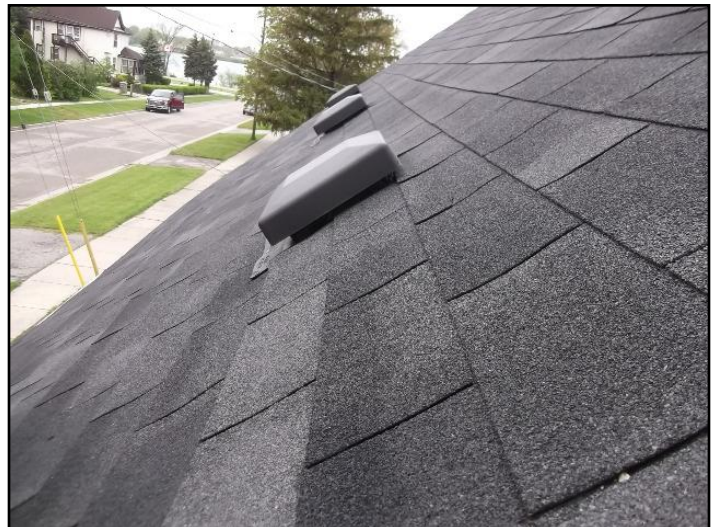
5. Asphalt shingles
