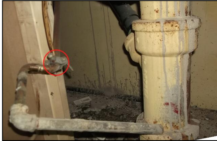
55. Wire attached to abandoned pipe
