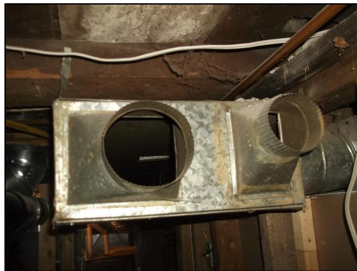
73. Disconnected ducts
