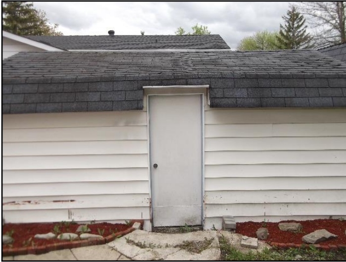
6. Asphalt shingles - west garage
