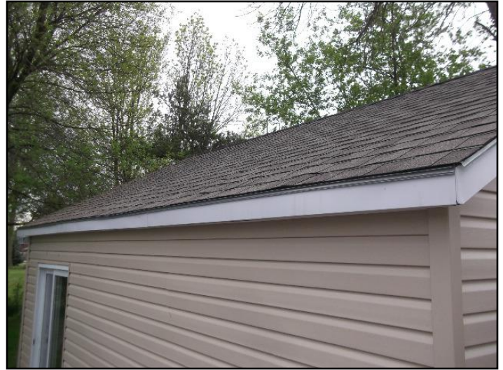
7. Asphalt shingles - east garage
