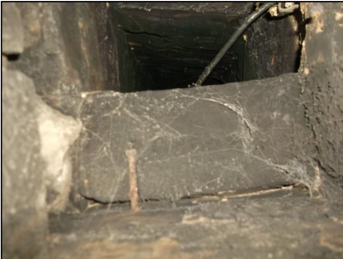
75. Open chimney flue
