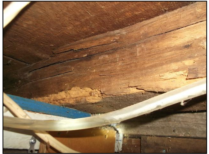
43. Damaged wood beam
