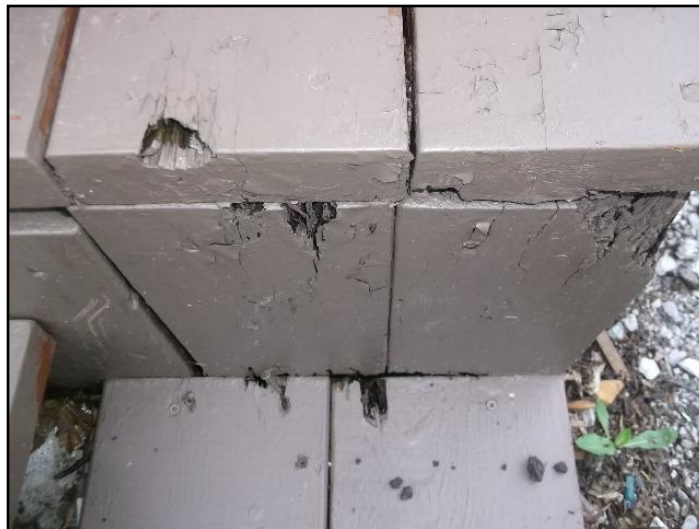
38. Rot or insect damage
