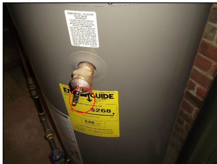
89. Discharge tube missing
