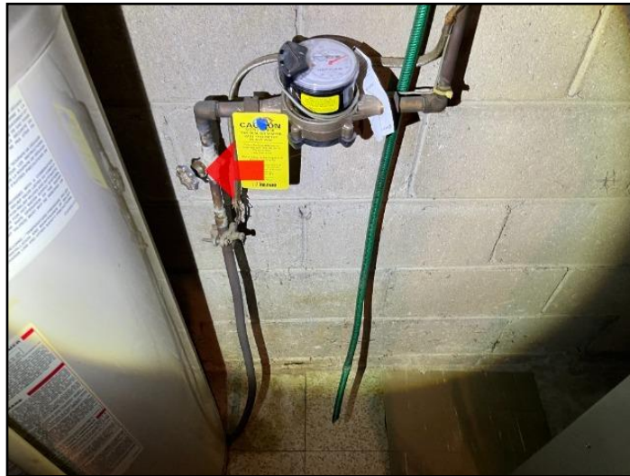
22. Main water shut off valve
