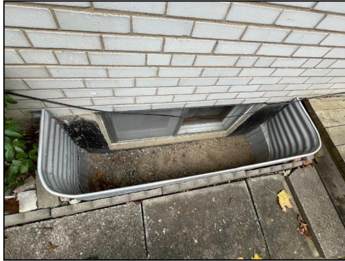
3. Less than 6 inches below window
