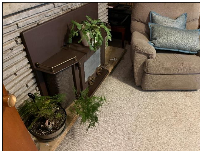
20. Floor - combustible clearance inadequate
