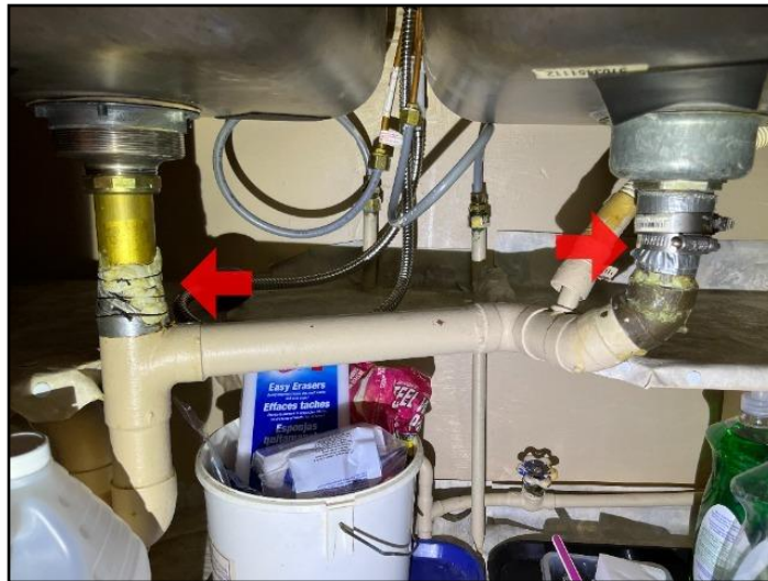
23. Nonstandard materials and patches
