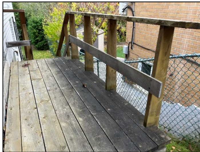
5. Spindles (balusters) climbable
