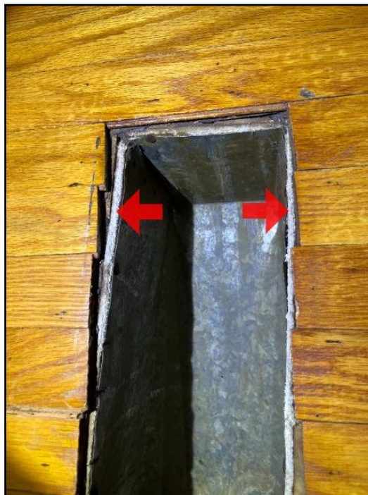
31. Possible asbestos containing materials
