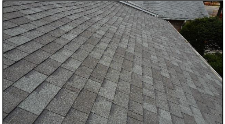
2. Asphalt shingles
