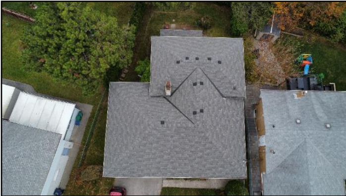
1. Asphalt shingles
